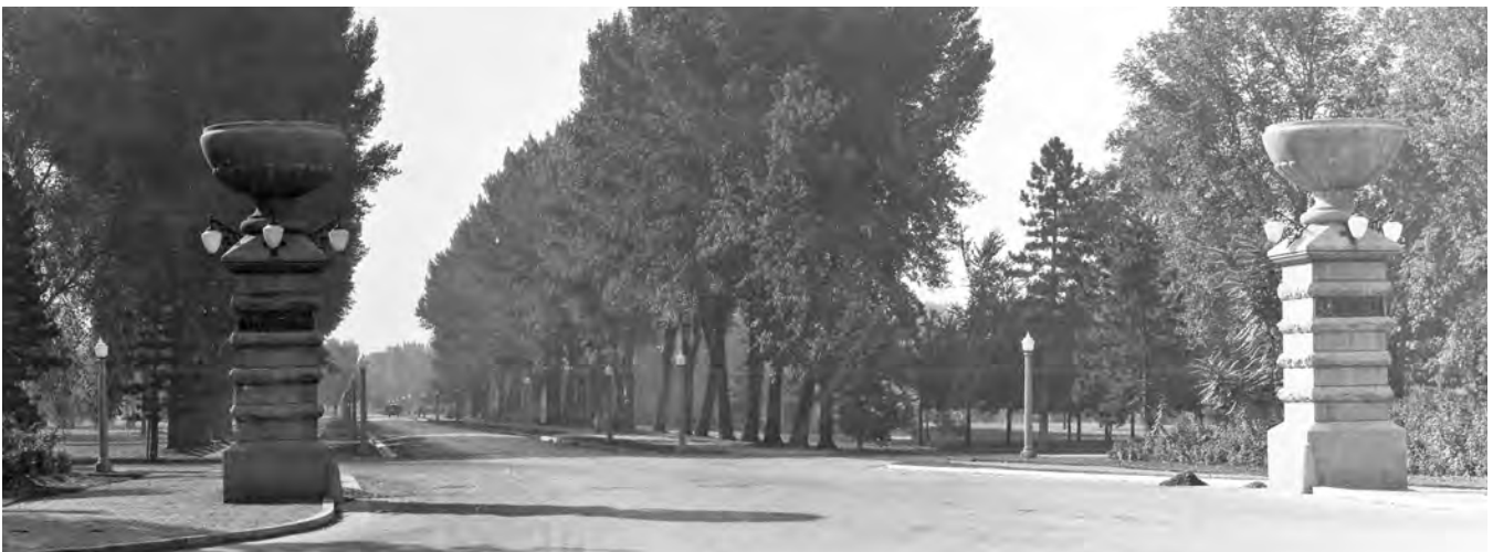
600 E after the addition monumental entrance piers, lights, curbs, and gutters, before 1918 (image: © Utah State Historical Society).
