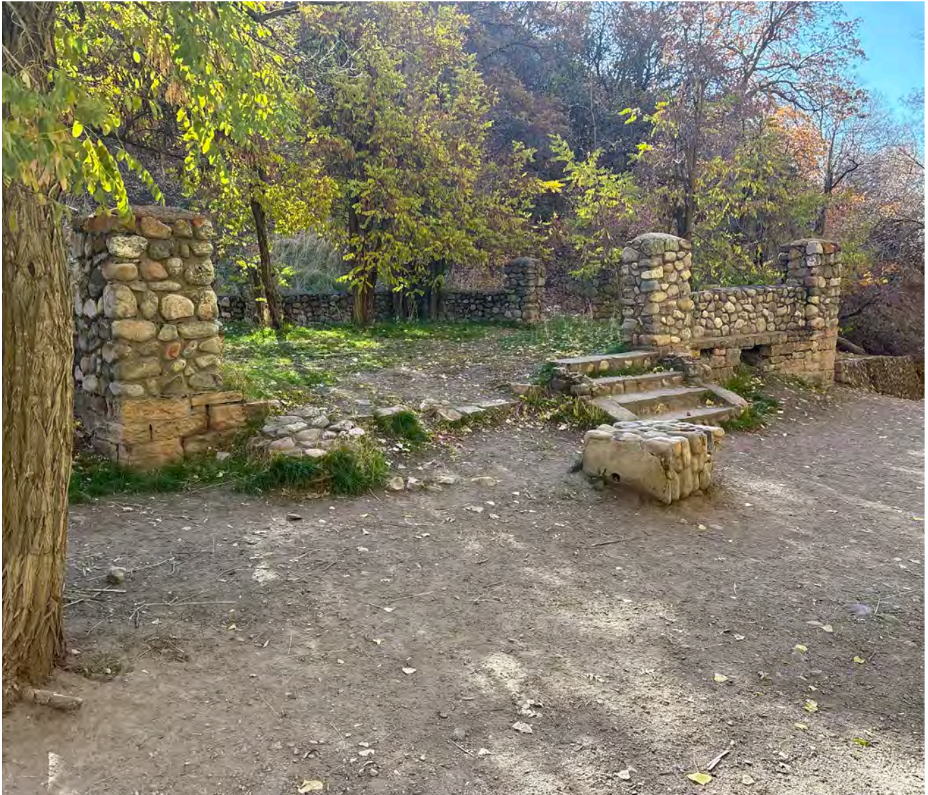
Figure 3-20. Foundations along Freedom Trail mark the location of the former Sundbury House and later rehabilitated as a bandstand (source top image: © Utah State Historical Society, 1950 and bottom image: Mundus Bishop, 2025).
