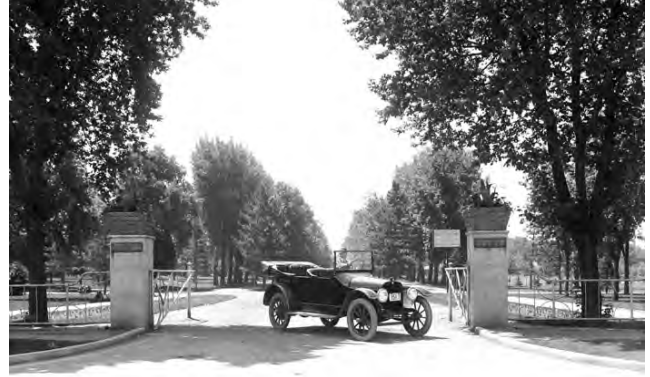
900 S park entrance with monumental entrance piers, 1915 (image: © Utah State Historical Society).
