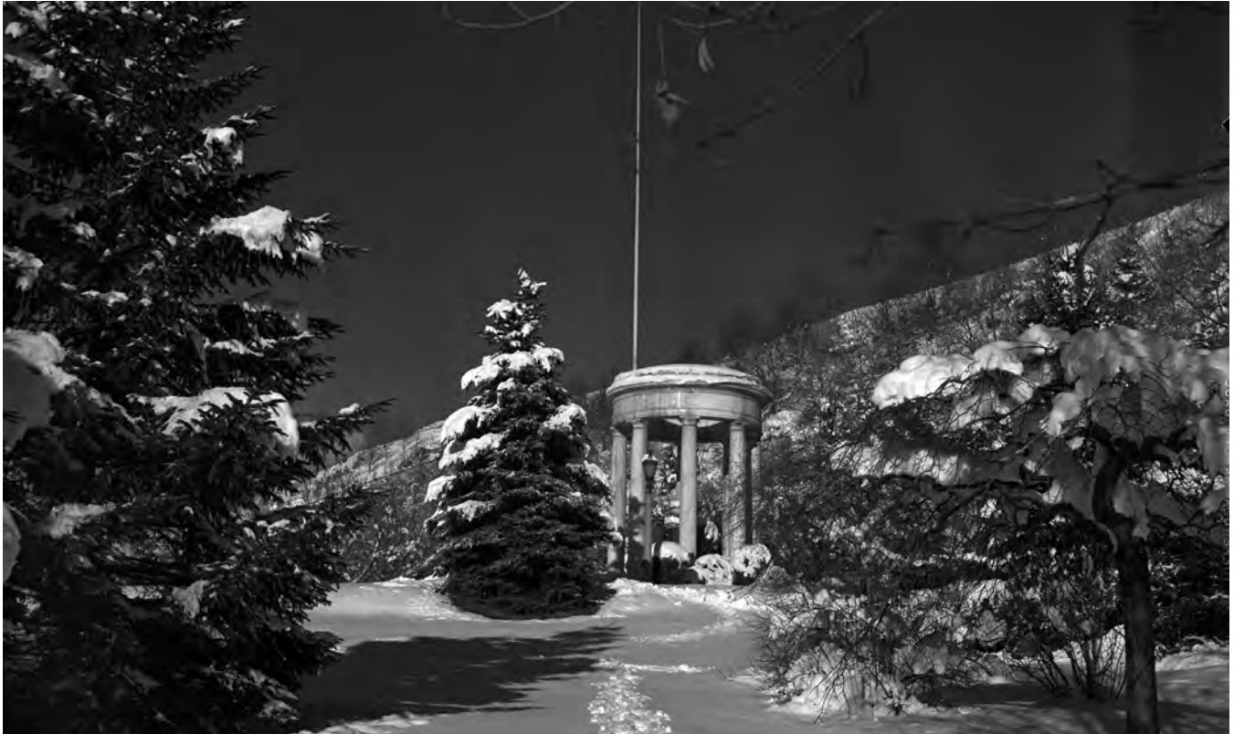
Figure 2-13. World War I Pagoda in 1939, looking northeast (source: © Utah State Historical Society).
