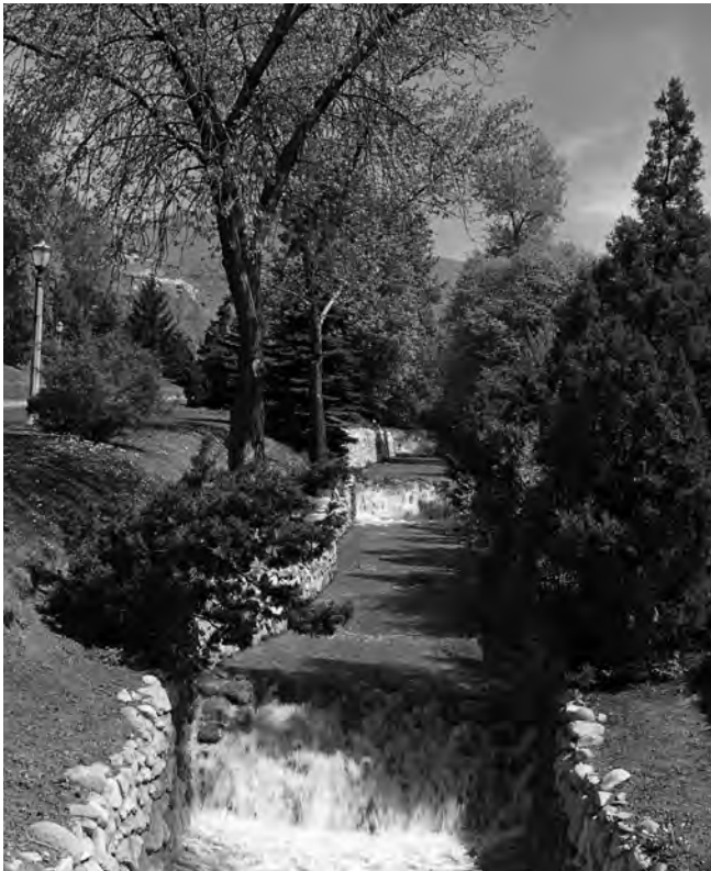
Figure 3-23. Stone drop structures and walls established during the period of significance remain along City Creek. Modifications include the addition of CMU block walls and replacement with concrete where impacted by previous flooding or to address erosion (source: historic images: © Utah State Historical Society; present-day images: Mundus Bishop, 2025).
