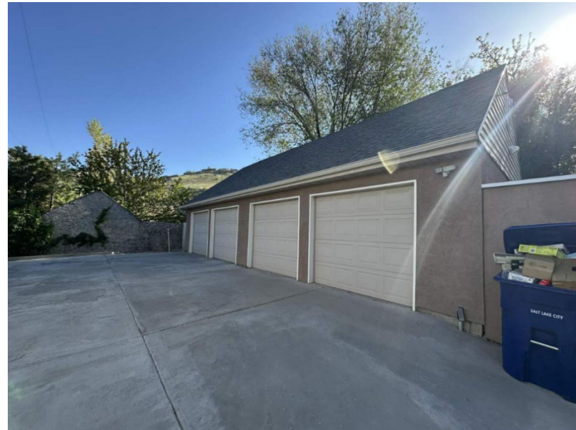
View of existing garage at the rear of the property, looking north
