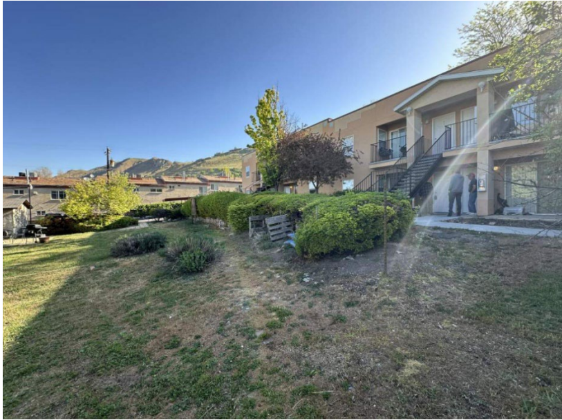
View of existing multifamily dwelling looking north/east.
