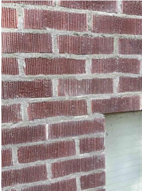
Example of similar brick condition at JOANN apartments after paint was removed. It was subsequently re-pointed. The mortar is does not match already appears to be coming off.
