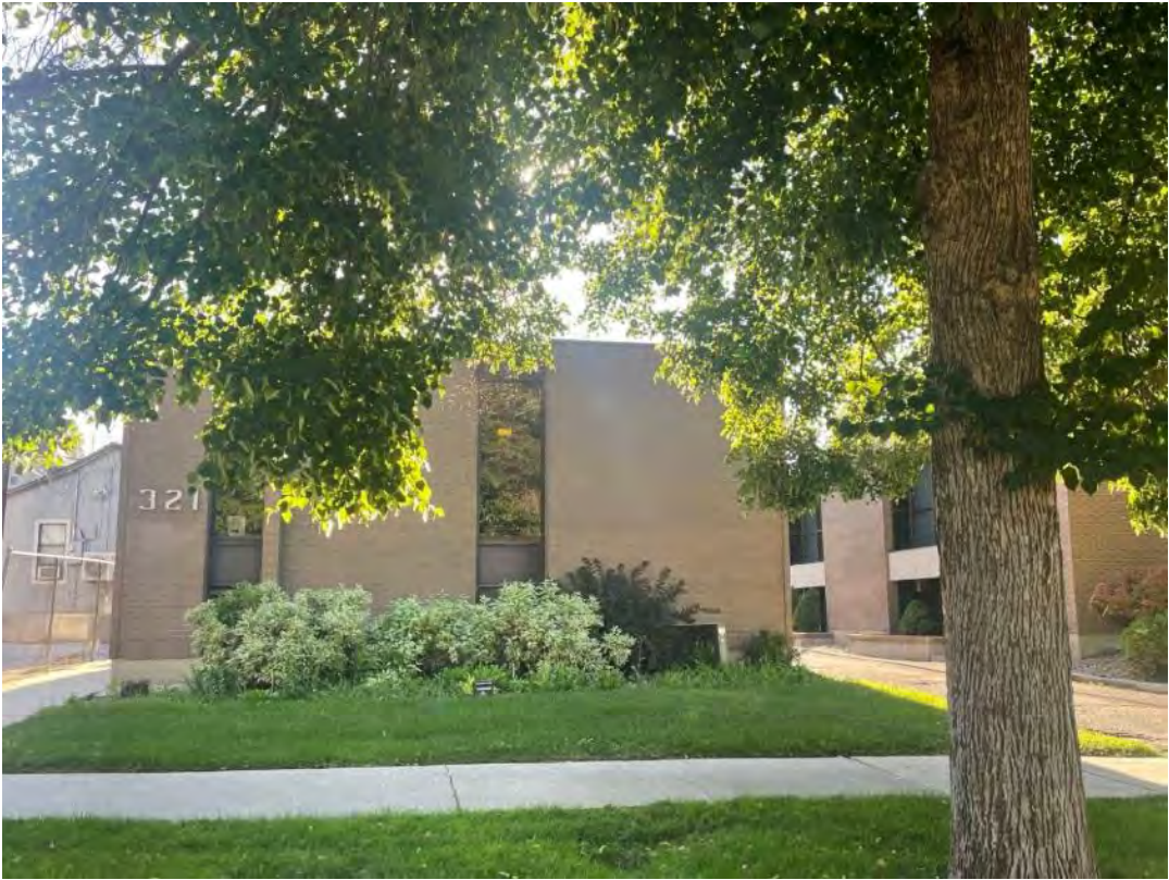
Existing structure at 321 S 600 E
