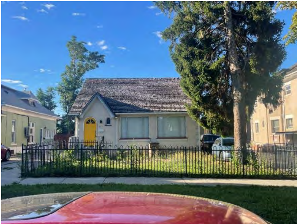
Existing structure at 612 E 300 S
