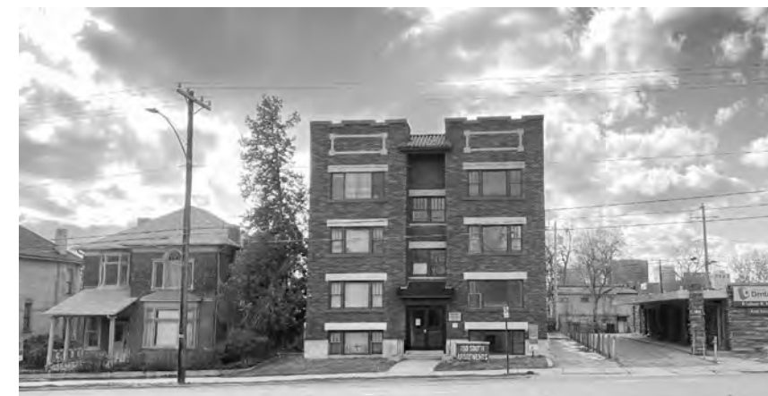
150 S 700 E LOCAL + NATIONAL CENTRAL CITY HISTORIC DISTRICT YEAR BUILT: 1927 3 STORY + BELOW GRADE BASEMENT
