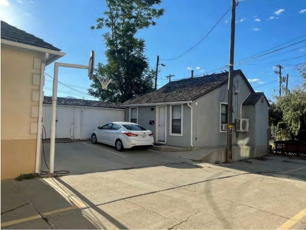
Existing structure at 614 E 300 S
