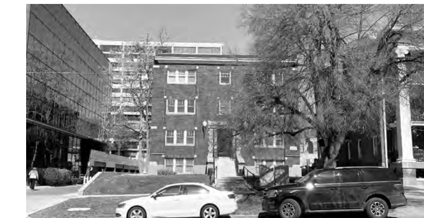
555 E 100 S LOCAL + NATIONAL CENTRAL CITY HISTORIC DISTRICT YEAR BUILT: 1928 3 STORY + BELOW GRADE BASEMENT
