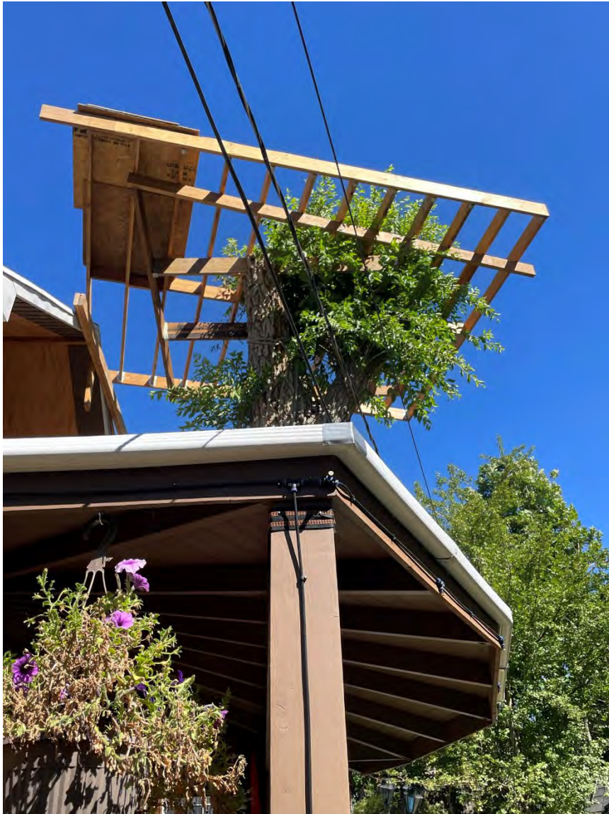
View of tree platform, facing north
