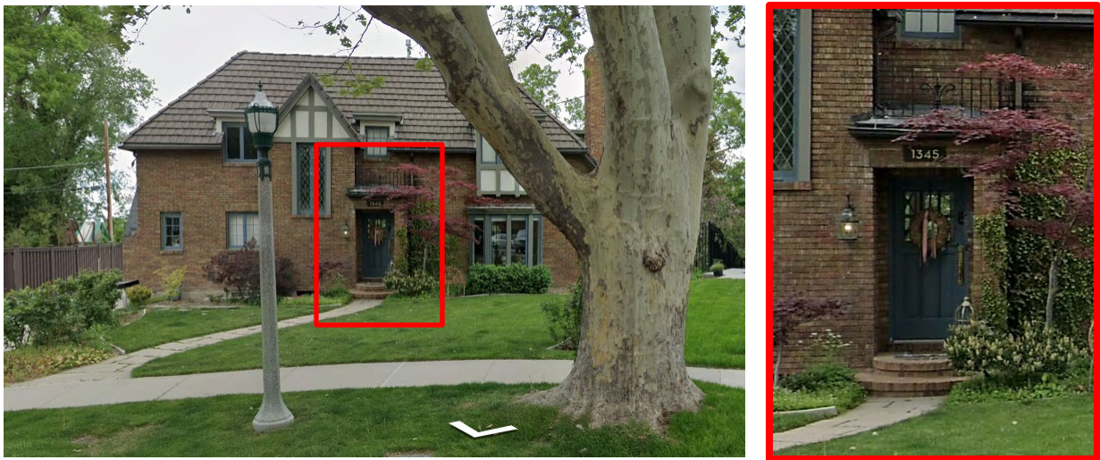
Figure 5 – Front of the house and close up of the porch prior to changes. The original steps were a distinctive feature and corresponded to the style of the historic house.
