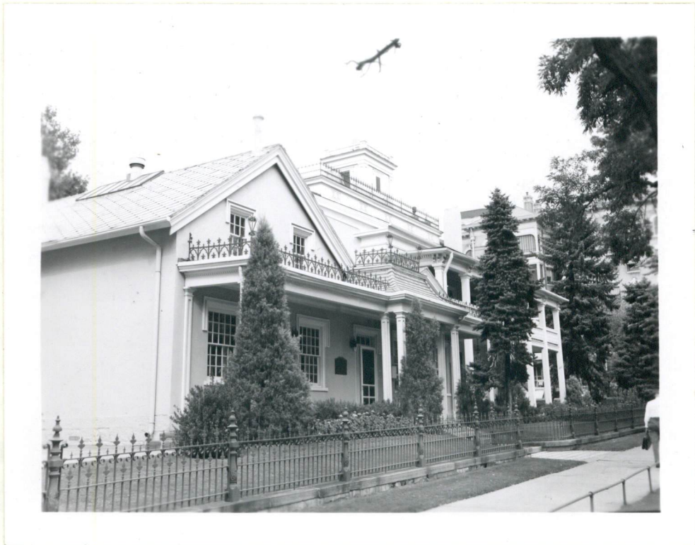
Lion House (left) and Beehive House, Salt Lake City, Utah. Photo by Robert M. Utley, Sept. 11, 1959. Negative in Region Three Office, National Park Service, Santa Fe, New Mexico.
