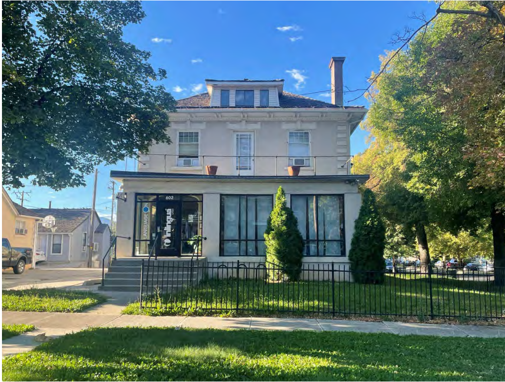
Existing structure at 602 E 300 S
