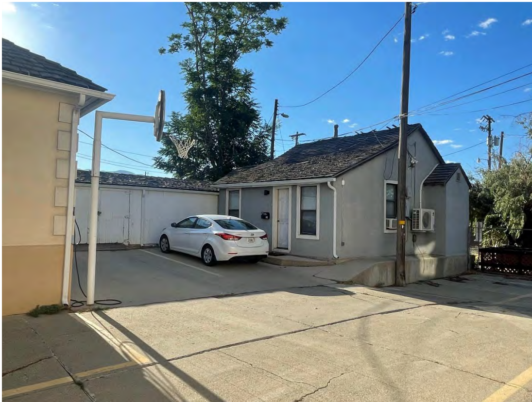
Existing structure at 614 E 300 S
