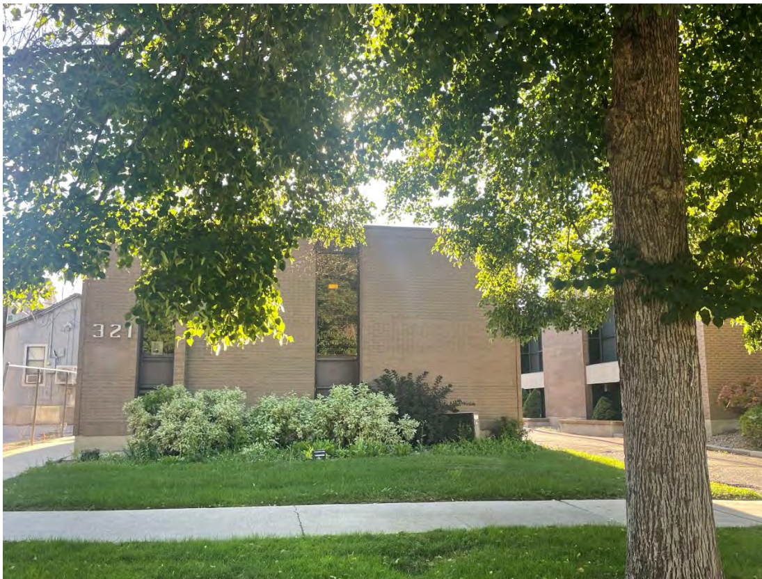
Existing structure at 321 S 600 E
