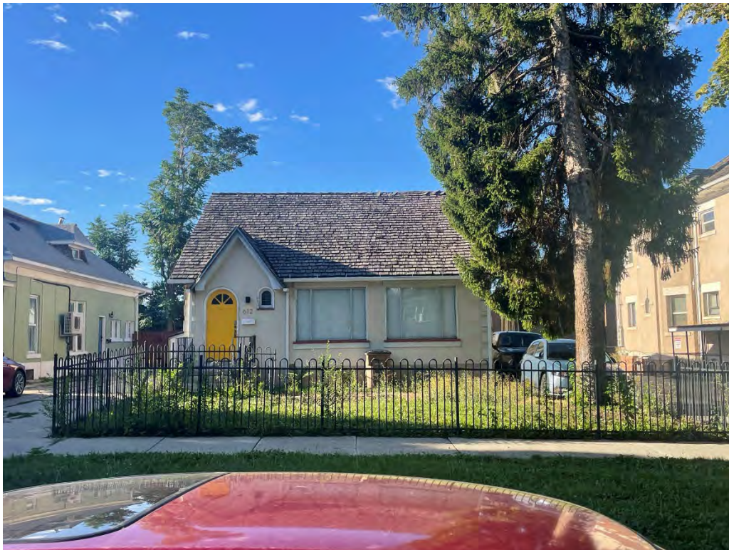
Existing structure at 612 E 300 S
