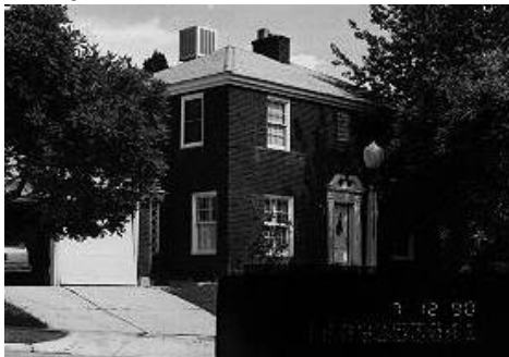
1425 E Laird Circle (A): 16-09-353-041 1939/35 Colonial Revival
