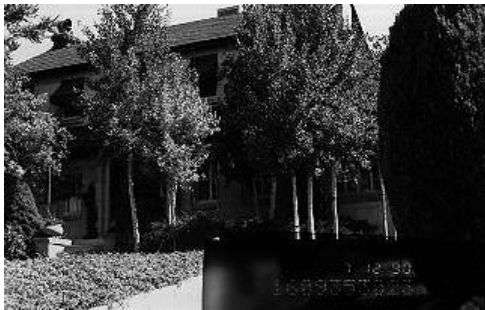
1417 E Laird Circle (B): 16-09-353-023 1931 Colonial Revival
