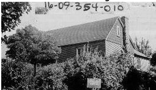
1380 E Laird Ave (B): 16-09-354-010 1927 Period Revival Cottage
