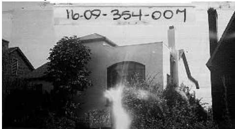
1362 E Laird Ave (A): 16-09-354-007 1927 Spanish Colonial Revival
