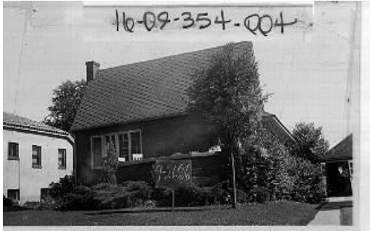
1342 E Laird Ave (A) 16-09-354-004 1927 Period Revival Other
