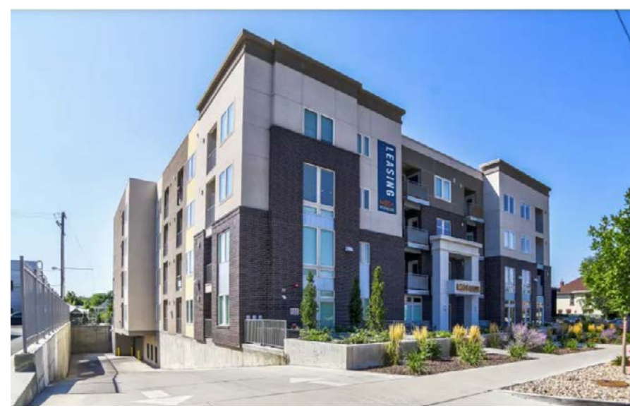
10 MODA NEWHOUSE APARTMENTS
