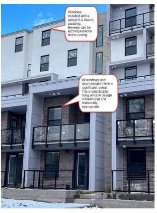
Good examples of appropriate windows installed in a recently approved multifamily development in a local historic district. These windows have been installed with a 2-3" reveal in a variety of façade claddings (brick, cementious panel, and stucco). Planning staff also notes the traditional style of the window and also notes that these windows are fibrex, a composite material.
