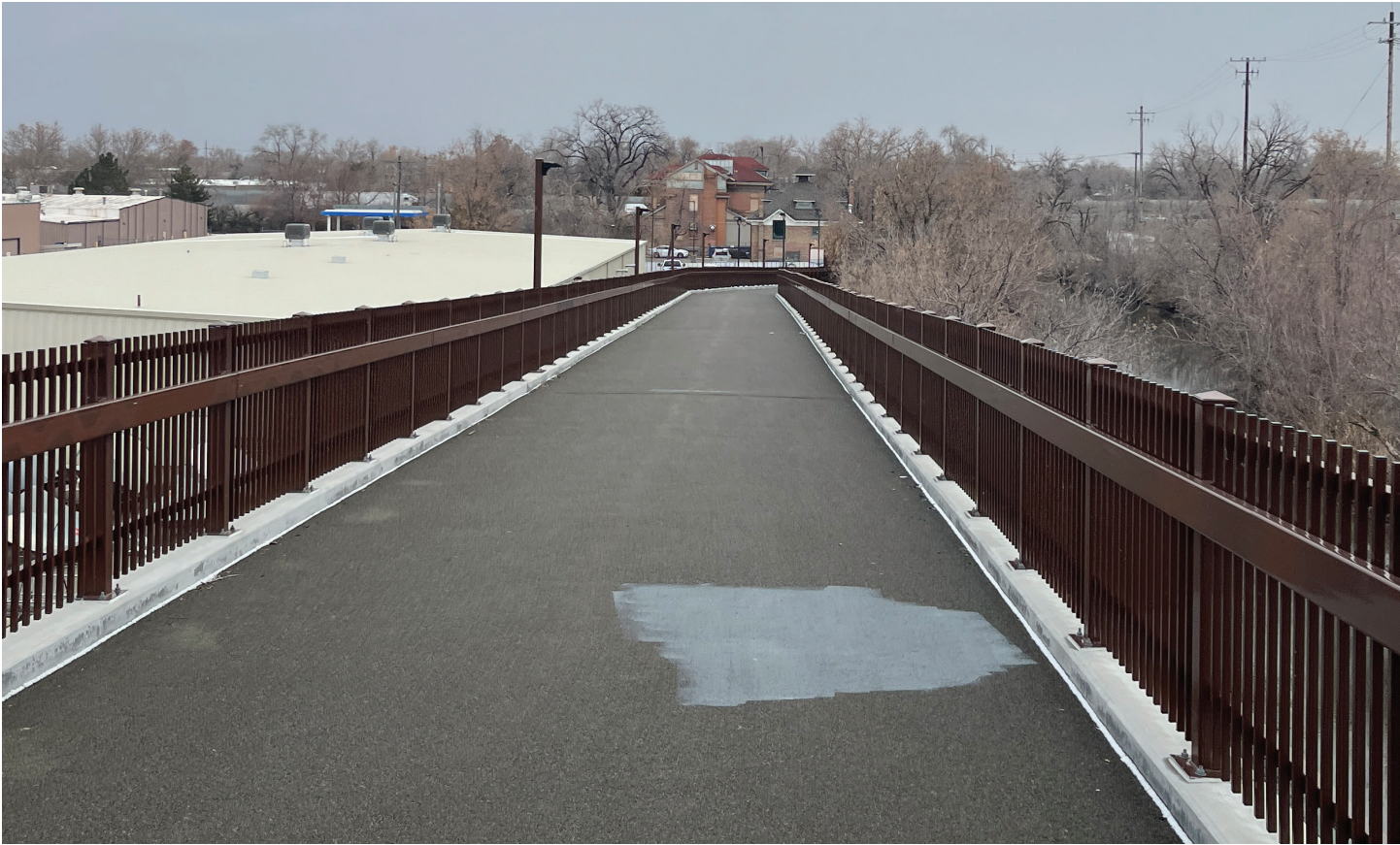
View 15 Looking S from point on bridge where Carriage House first comes to view
