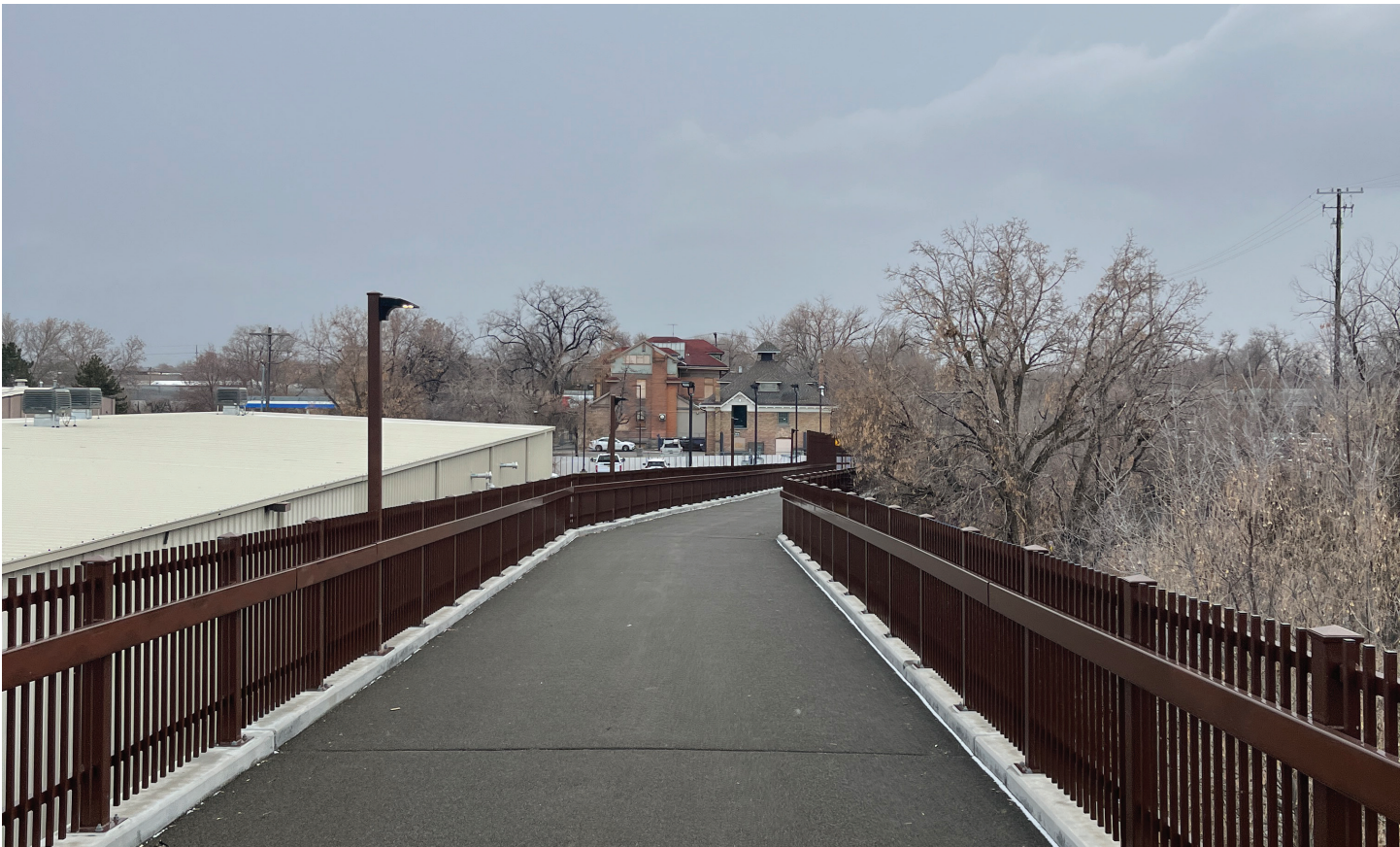
View 14 Looking S from further up bridge ascent
