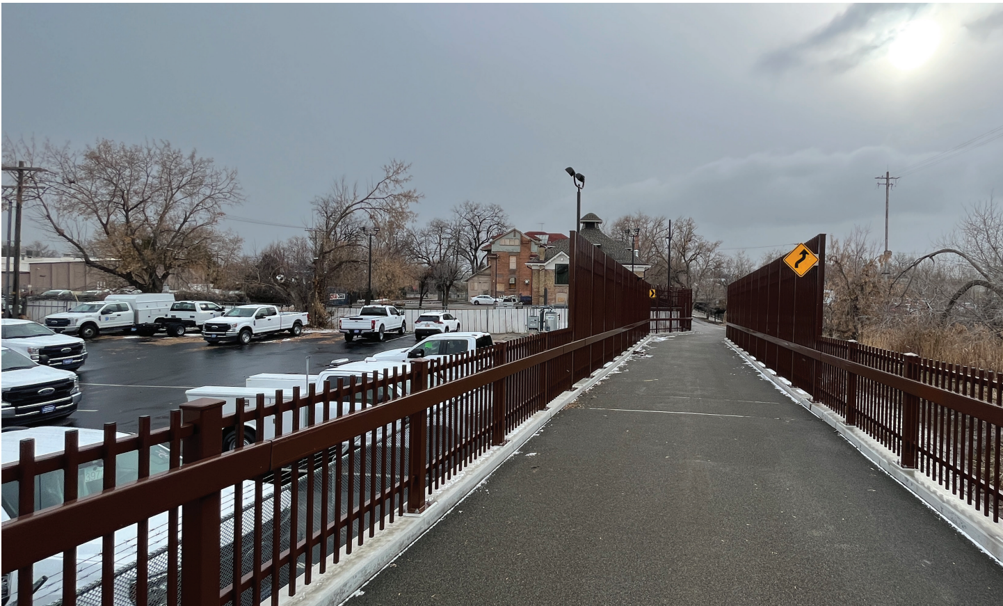
View 13 Looking S from further up bridge ascent
