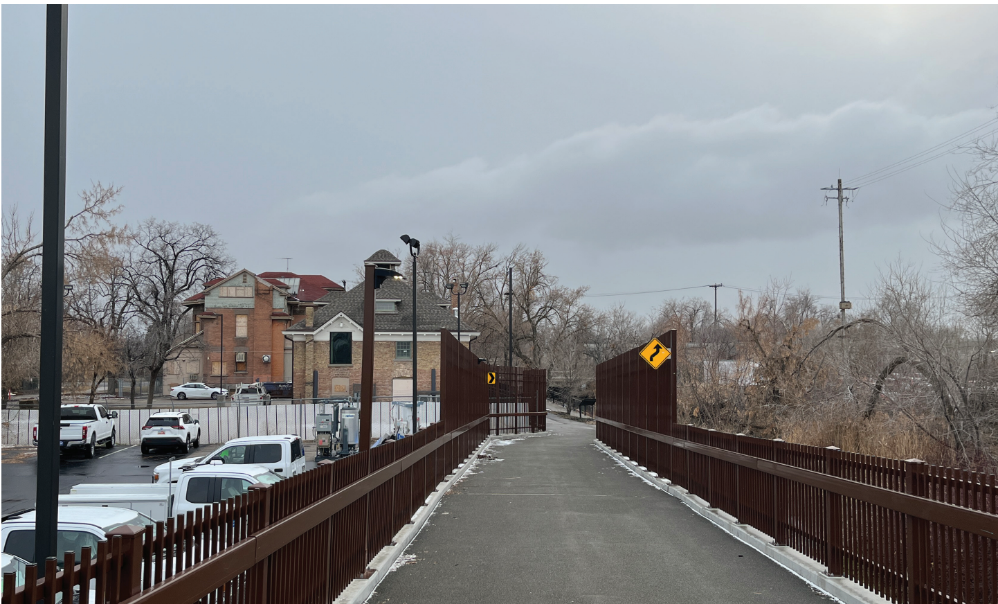
View 3 - Current painted conduit covers
