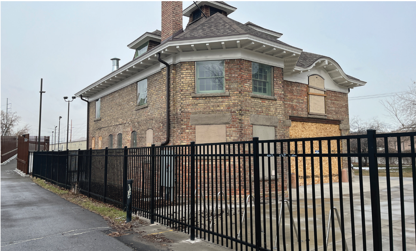
View 7 Looking NE while approaching Carriage House from trail
