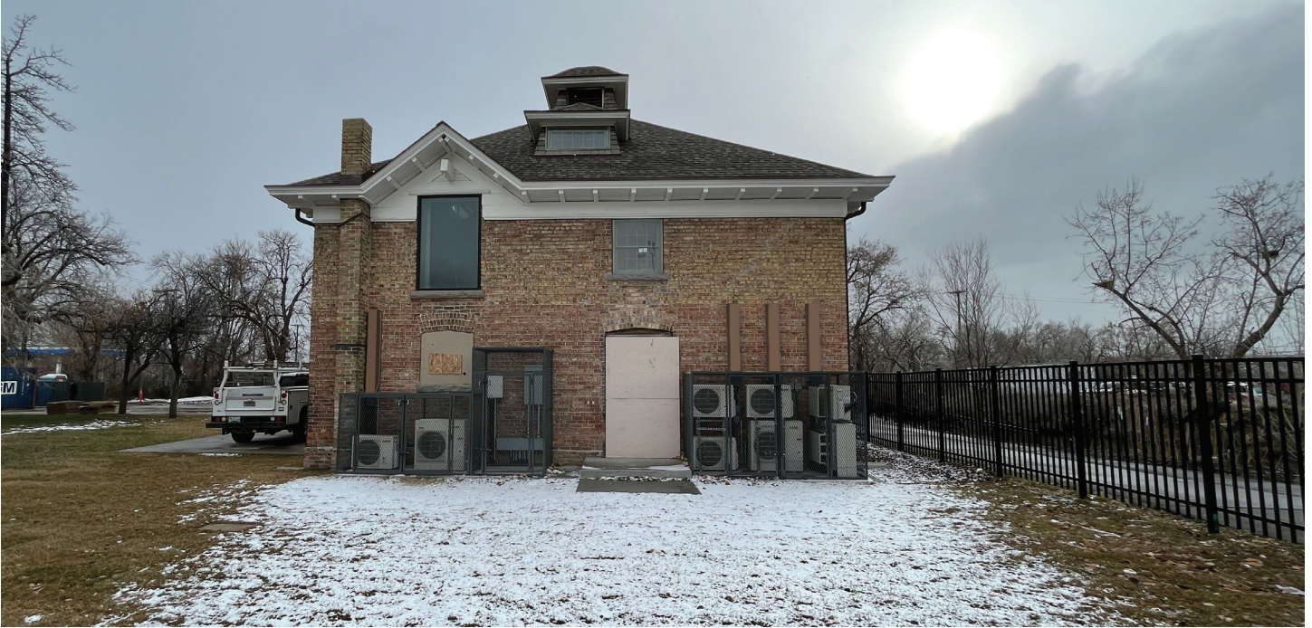
View 1 - Proposed painted conduit covers
