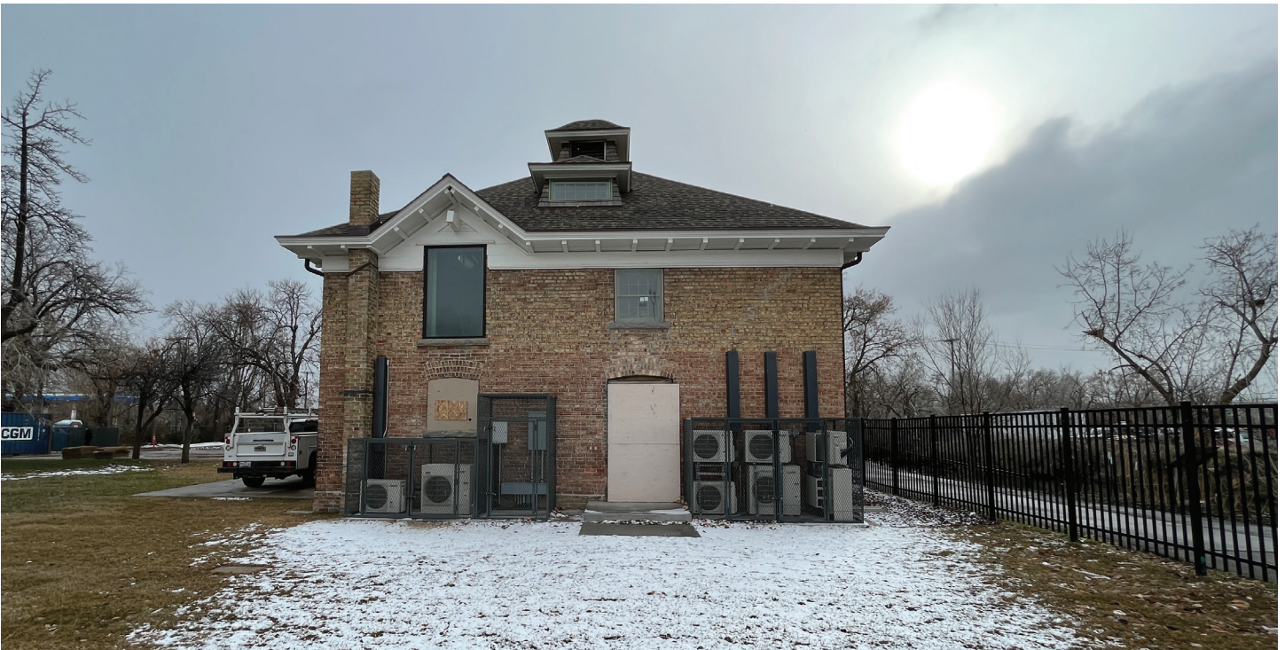
View 1 - Current painted conduit covers
