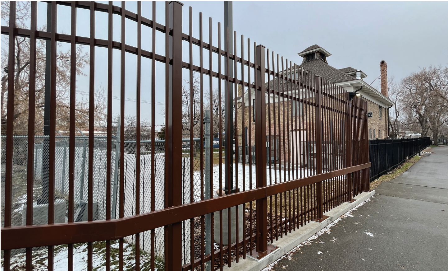
View 11 Looking SE from trail as starting bridge ascent
