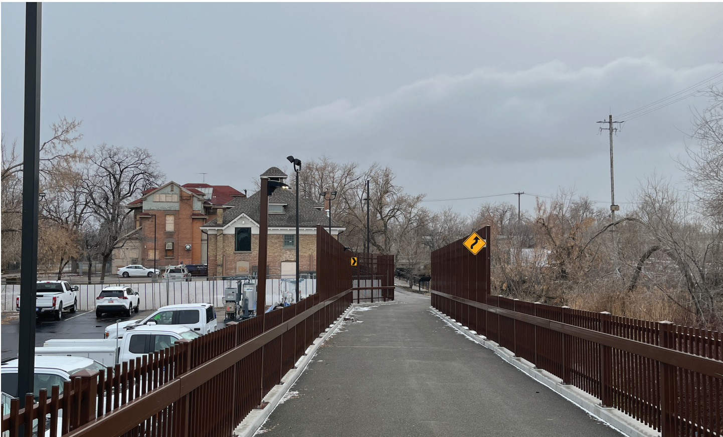
View 3 - Proposed painted conduit covers
