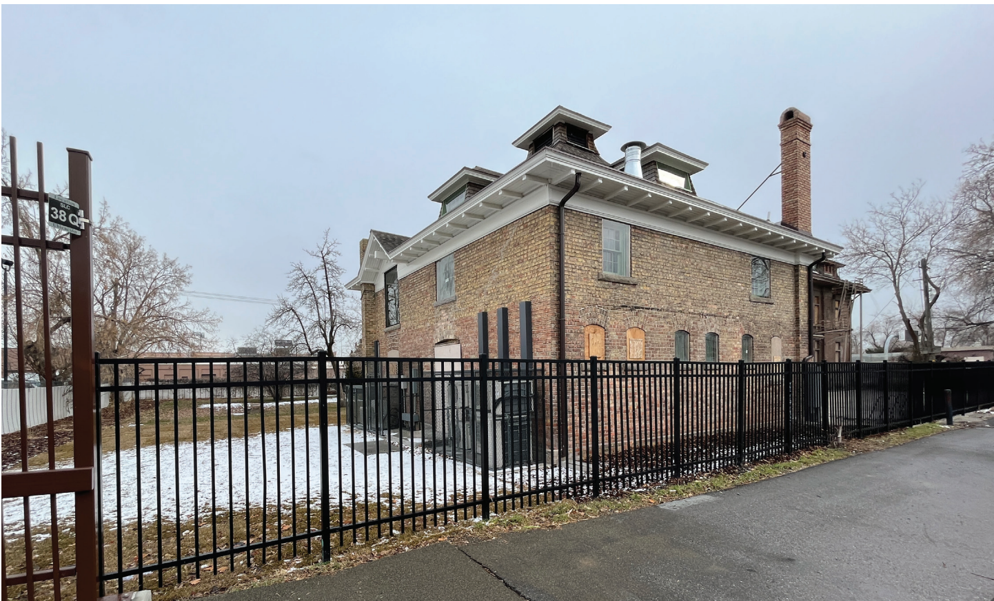
View 2 - Current painted conduit covers
