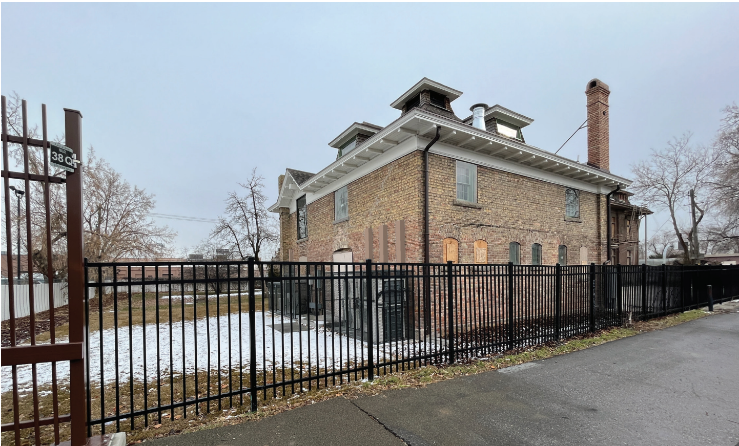
View 2 - Proposed painted conduit covers
