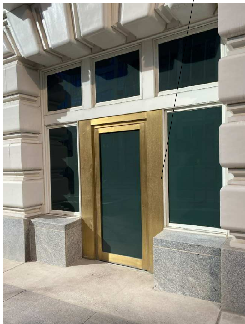
EXISTING EXIT DOOR
