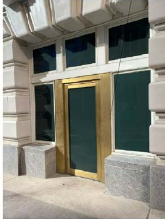
EXISTING EXIT DOOR
