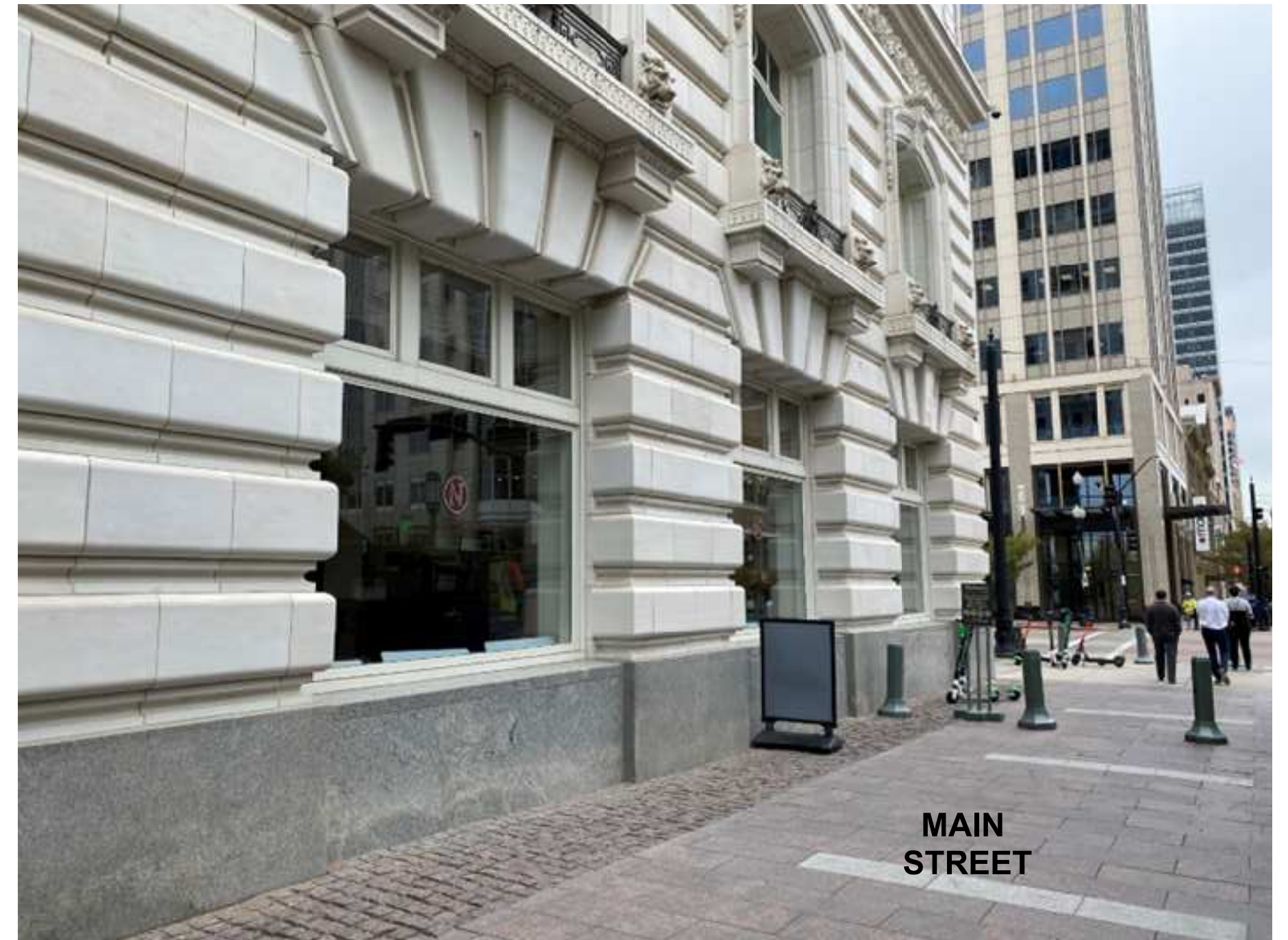
PHOTO SHOWING EXISTING CONDITION
