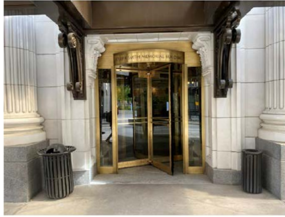
EXISTING REVOLVING DOOR
