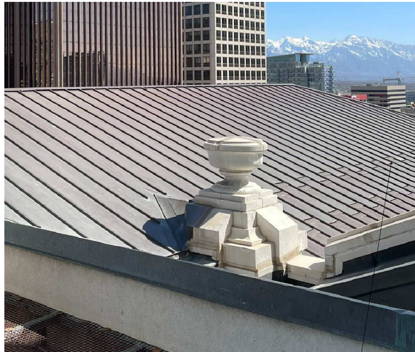
CURRENT ROOF PHOTO
