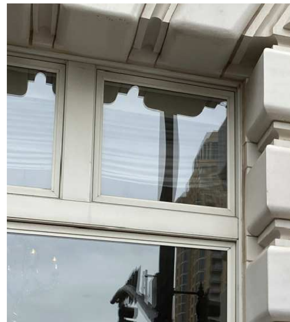
EXISTING WINDOW FRAMES
