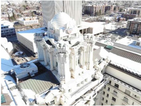
Existing Roof Conditions
