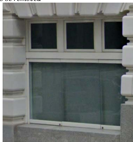
Replacement windows- added in 1993
