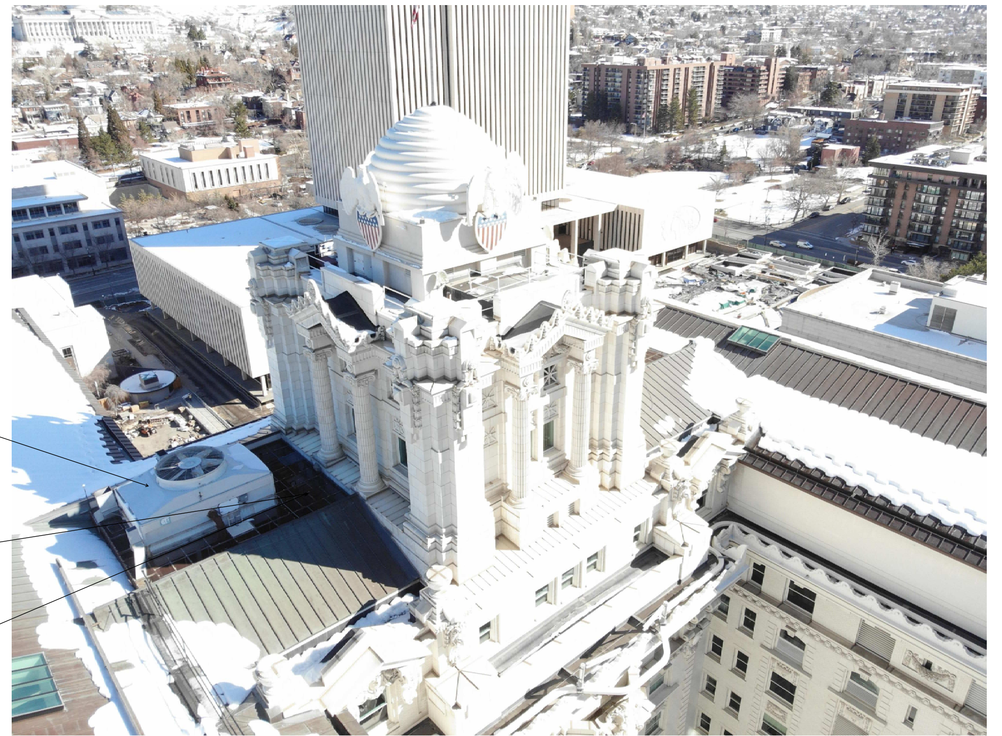
PHOTO SHOWING EXISTING CONDITION
