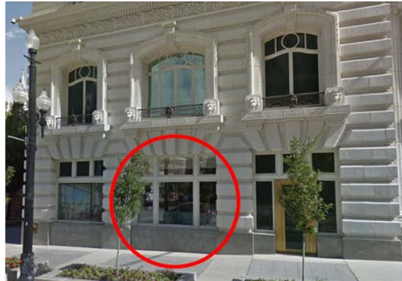
Existing Conditions - South Temple
