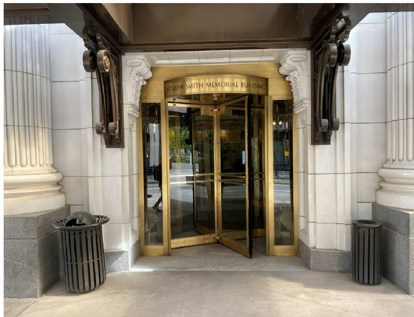
EXISTING REVOLVING DOOR
