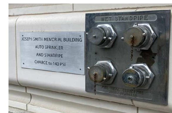
RELOCATED FIRE DEPT. CONNECTION
