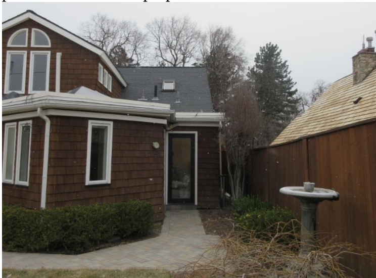
Rear façade, 1551 Sherman.
