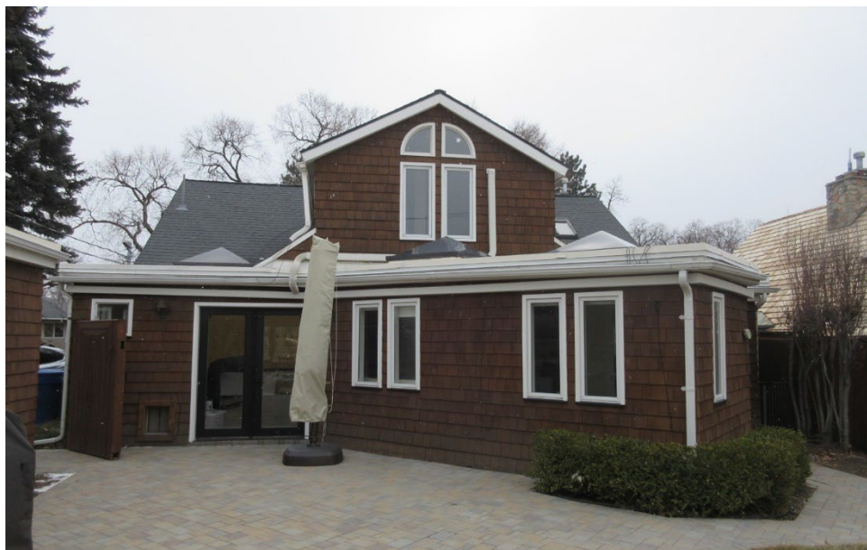
Rear façade, 1551 Sherman.
