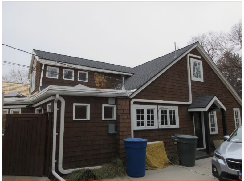
Historic House – East Facade
