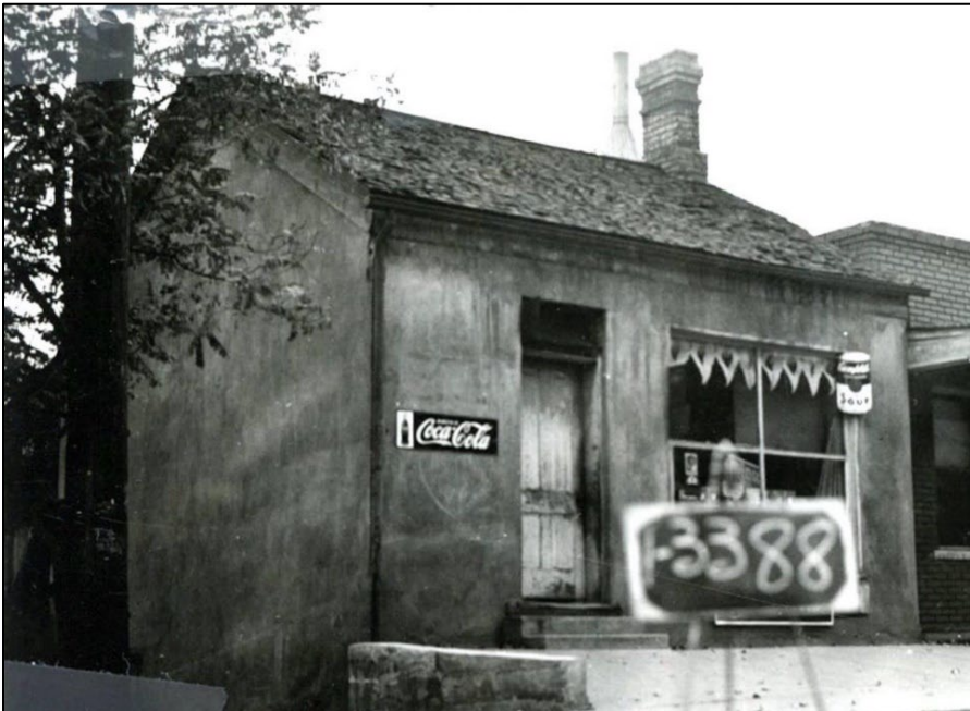
South and East elevation – front façade, historic photo from approximately 1936
