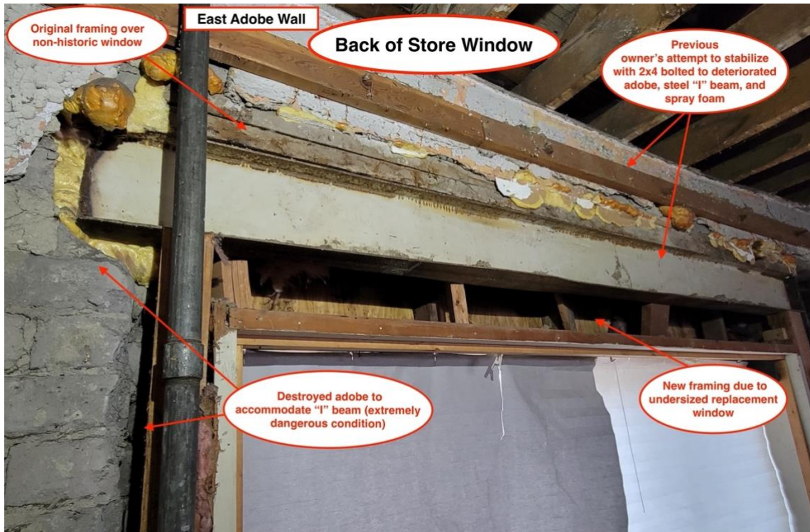
Main floor - east wall deterioration of adobe around missing transom window
