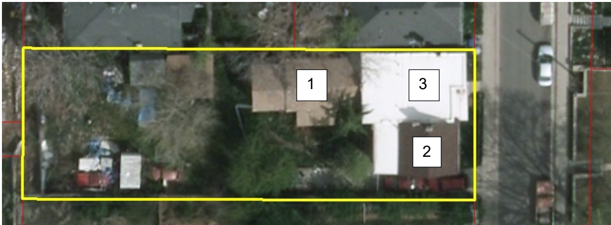
Aerial View – aerial view of the property with the three structures
