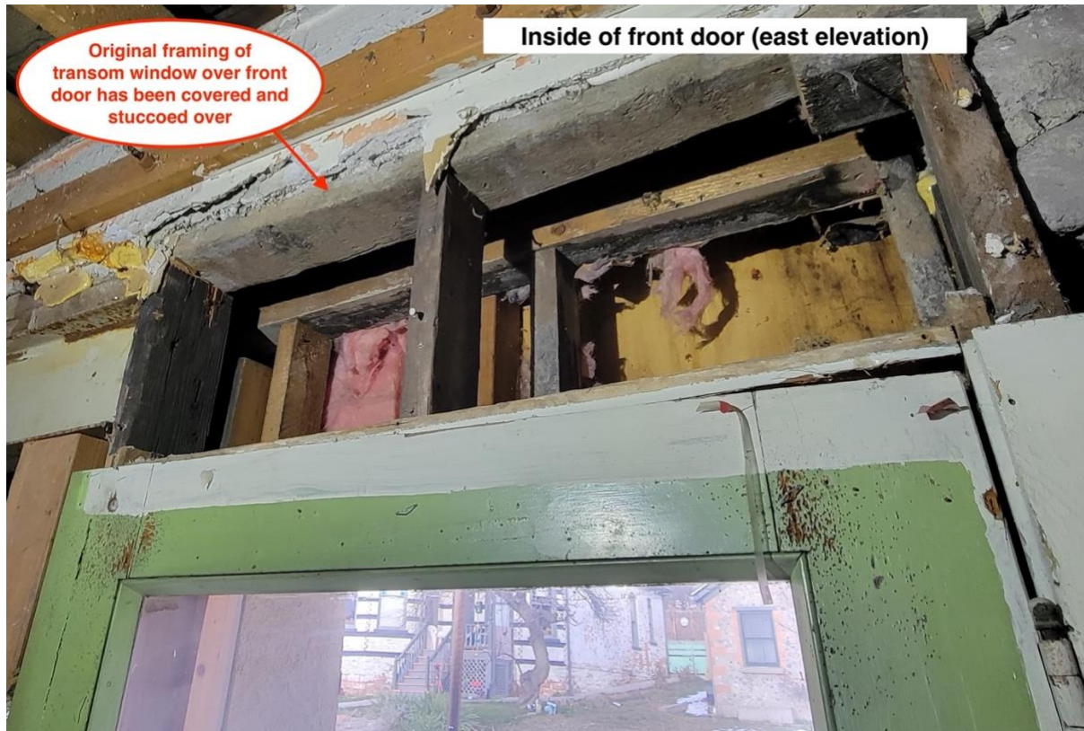
Main floor - east wall deterioration of adobe around missing transom window
