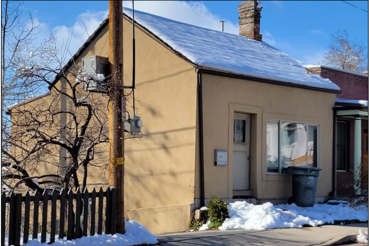
South and East elevation – front façade, current view
