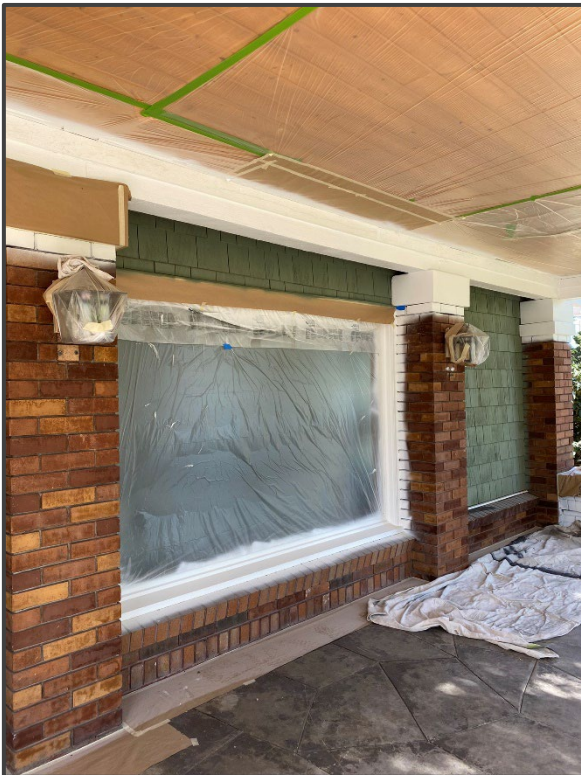
Left: Front wall before masonry was painted
