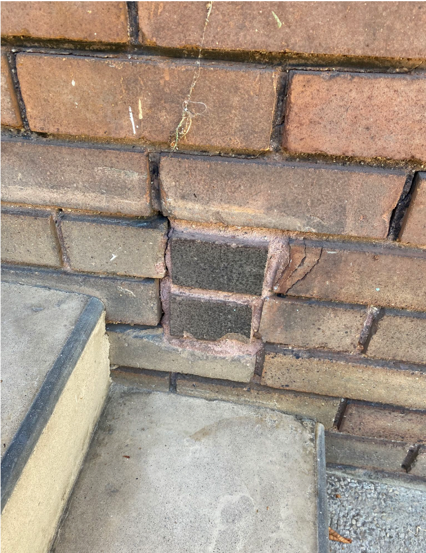
Another example of repaired brick with different color scheme
