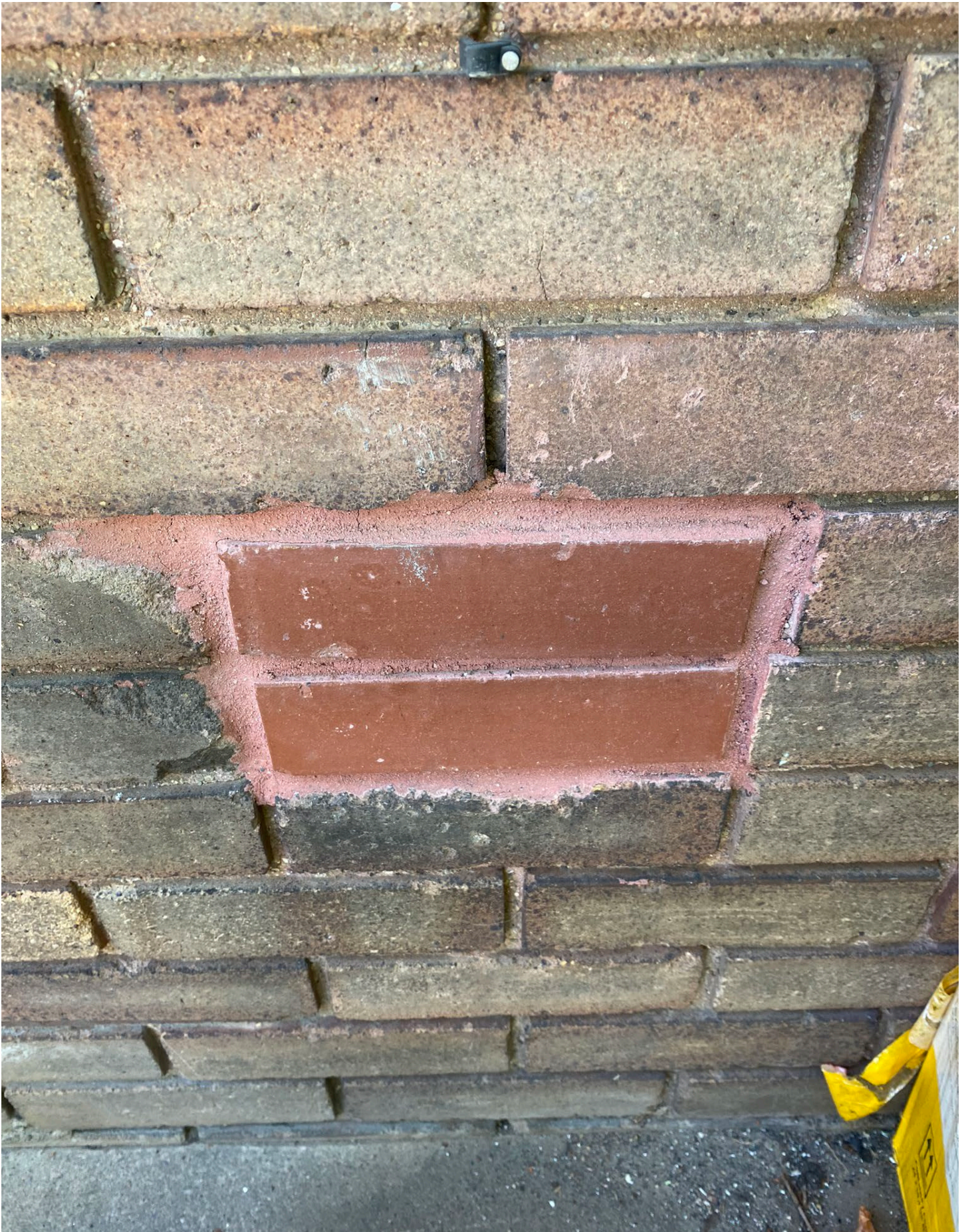
Example of repaired brick with different color scheme
