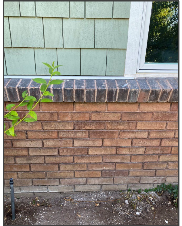
Detail view of unpainted brick
