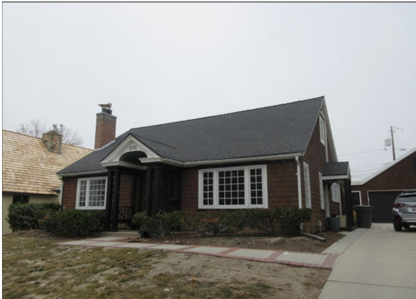
Subject Property – Front Facade
