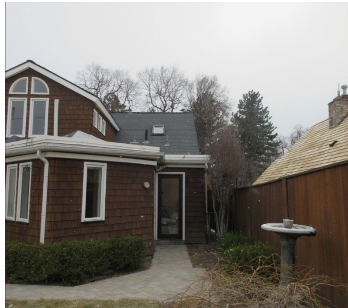
Historic House – Rear Façade (north-east)
