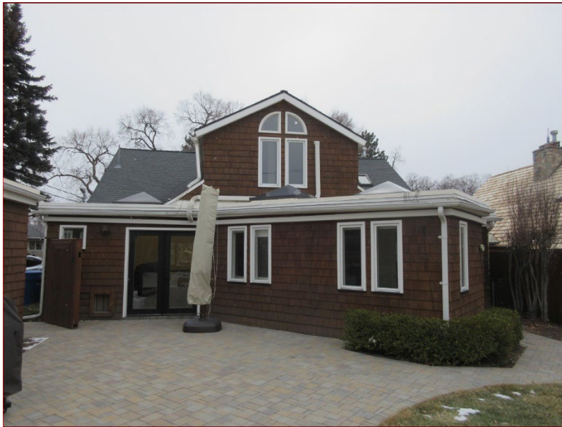
Historic House – Rear Façade (north)
