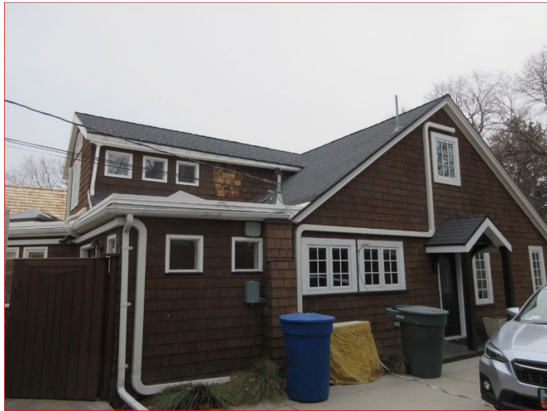
Historic House – East Facade
