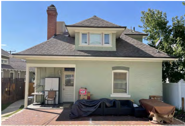
West Elevation – showing from the rear of the home the proposed chimney to be removed
