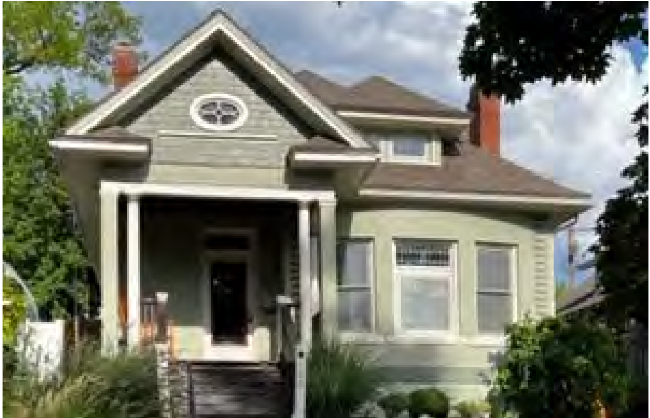
West Elevation - Street View showing two front chimneys (not showing proposed chimney to be removed)
