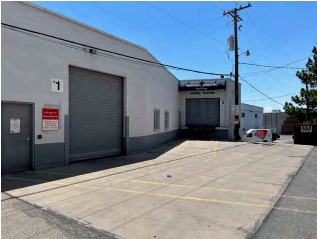
Modern Display warehouse buildings on Fuller Avenue.
