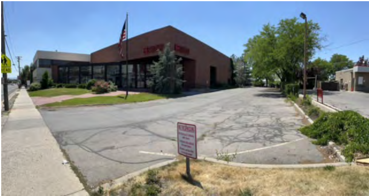
Modern Display Building on 700 East.
