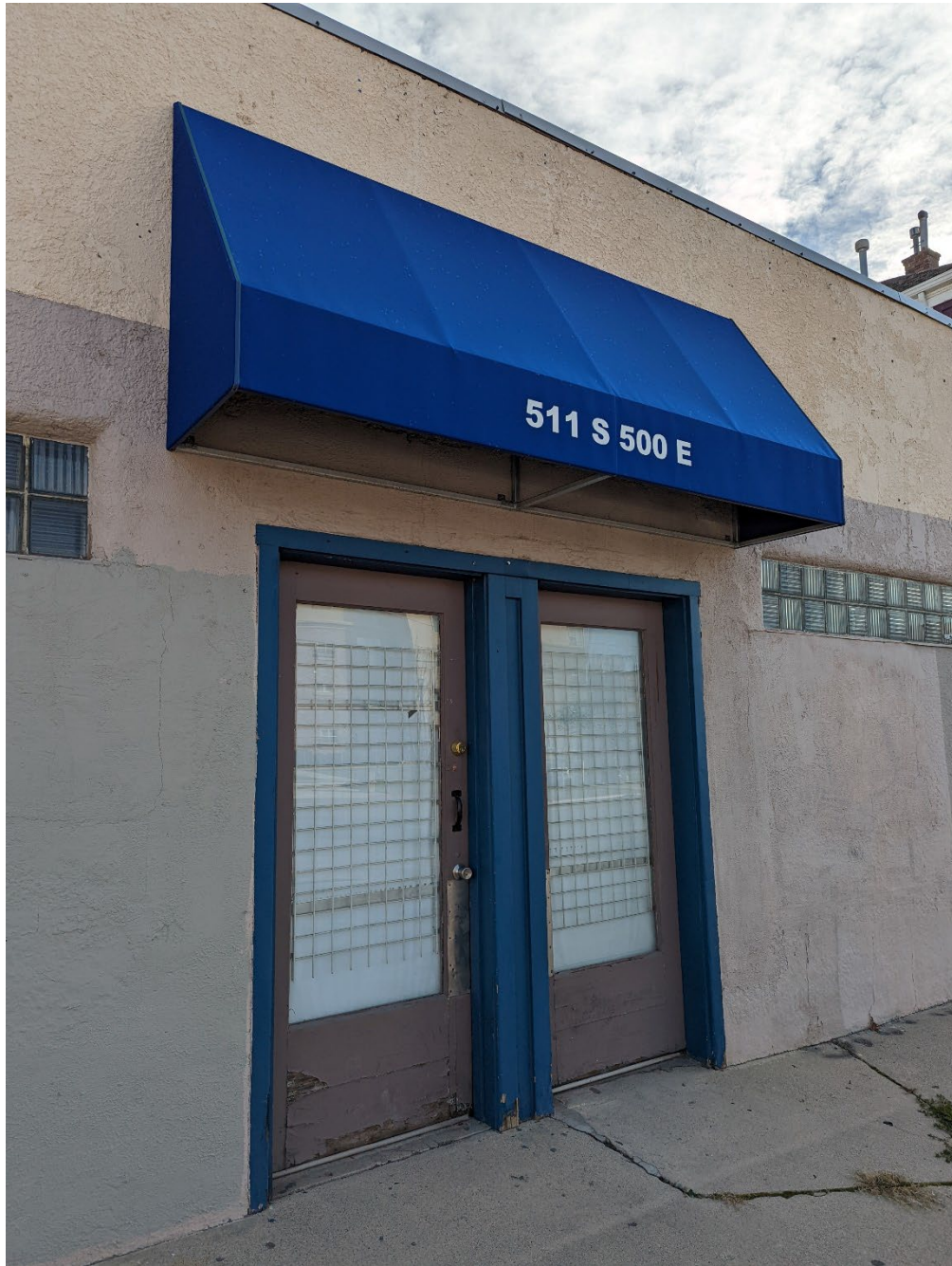
Figure 15: Entry Doors on West Elevation
