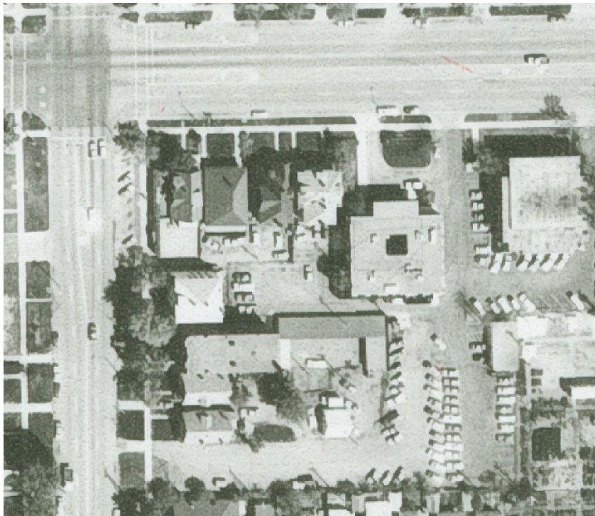
Figure 23: Aerial Image of Site and Surrounding Properties, 1985. Source: Utah Aerial Imagery Database, Utah Geologic Survey
