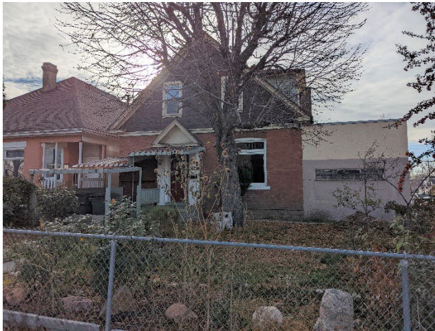
Figure 9: View of North Elevation
