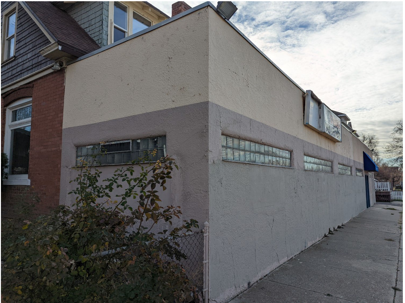
Figure 14: Closeup of North and West Elevations
