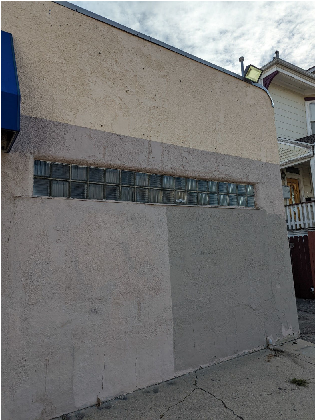
Figure 16: Glass block window on West Elevation
