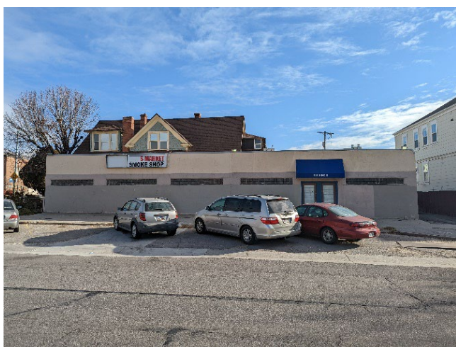
Figure 7: View of West Elevation
