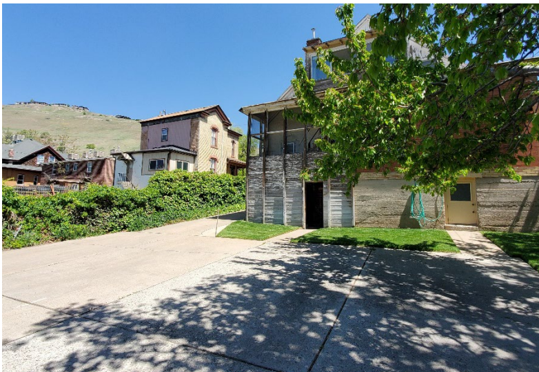
Rear (west) view – the lot slopes down towards the west as seen in the photo
