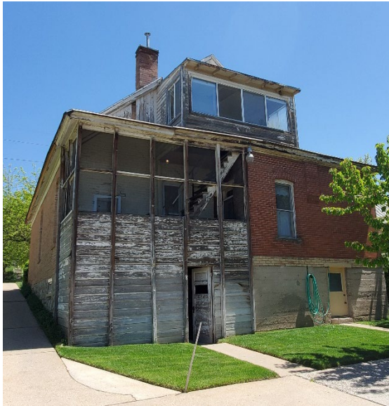
Rear (west) view of subject property
