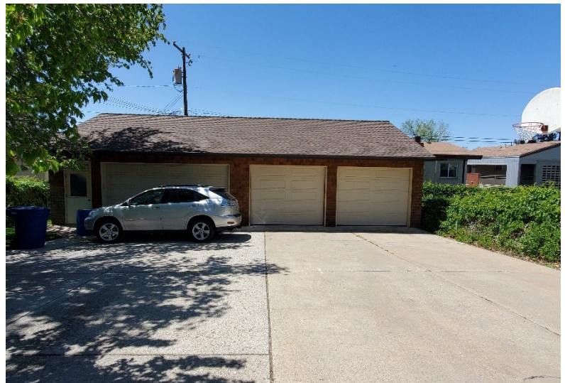
Existing garage in rear portion of subject property
