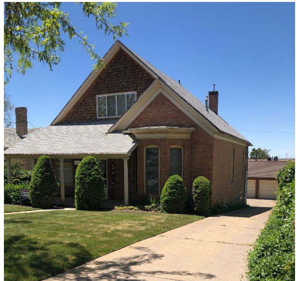
Sidewalk view of side of property from the north east corner
