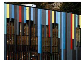
FIBRE C GLASS FIBRE REINFORCED CONCRETE PANELS
