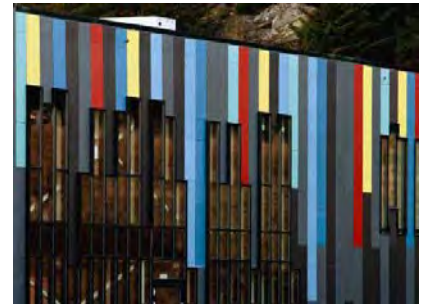
Figure 5 - GFRG Panels at north entrance
