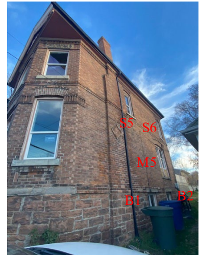
Figure 4: Western (side) façade
