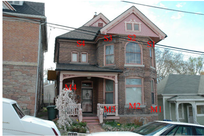
Figure 5: 2006 RLS Survey photograph of subject property showing original windows and woodwork details.
