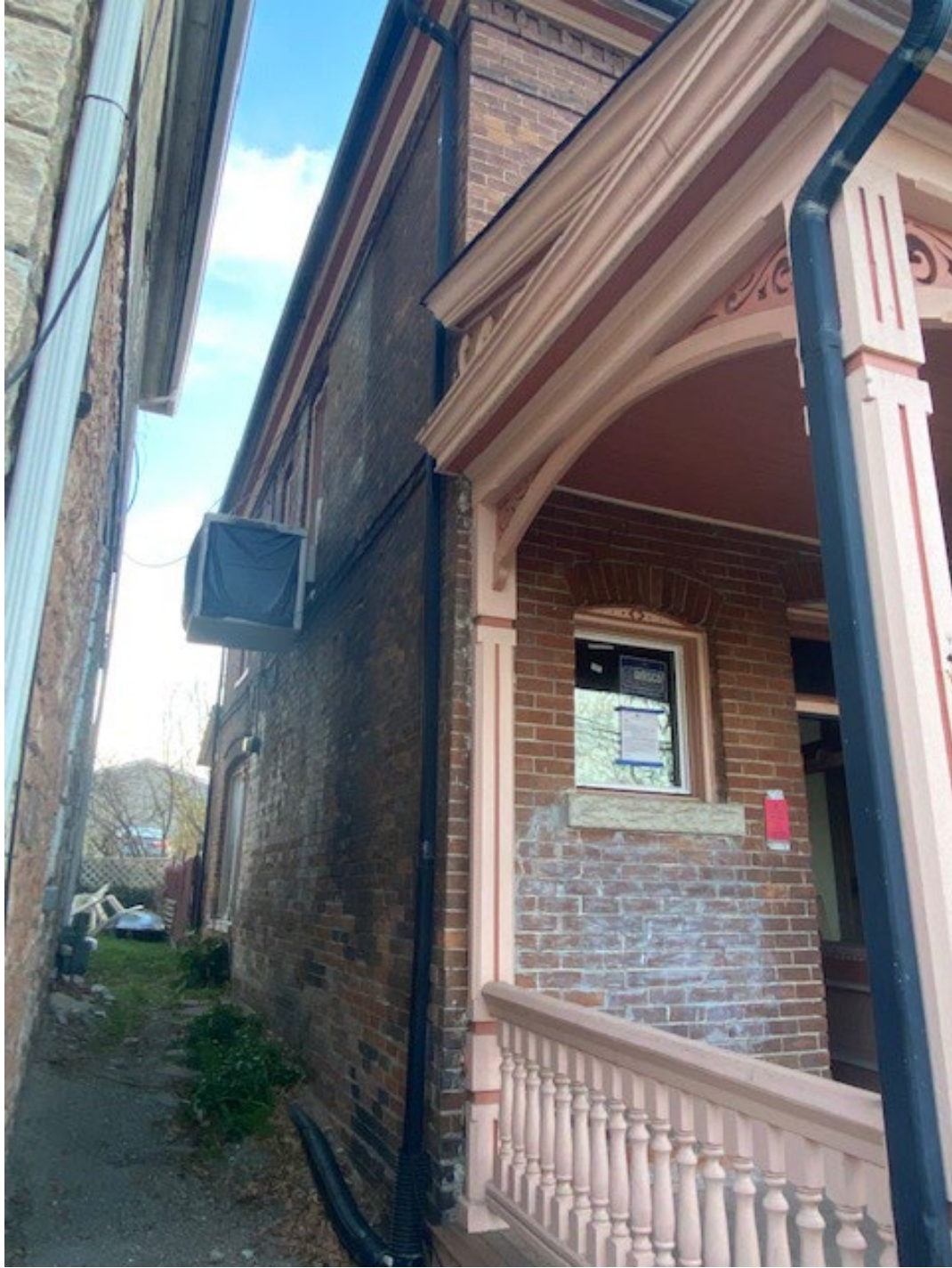
Figure 9: Photograph of side (eastern) facade provided by Applicant.
