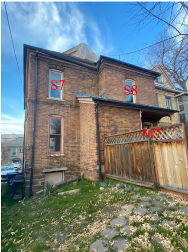
Figure 2: Southern (rear) façade
