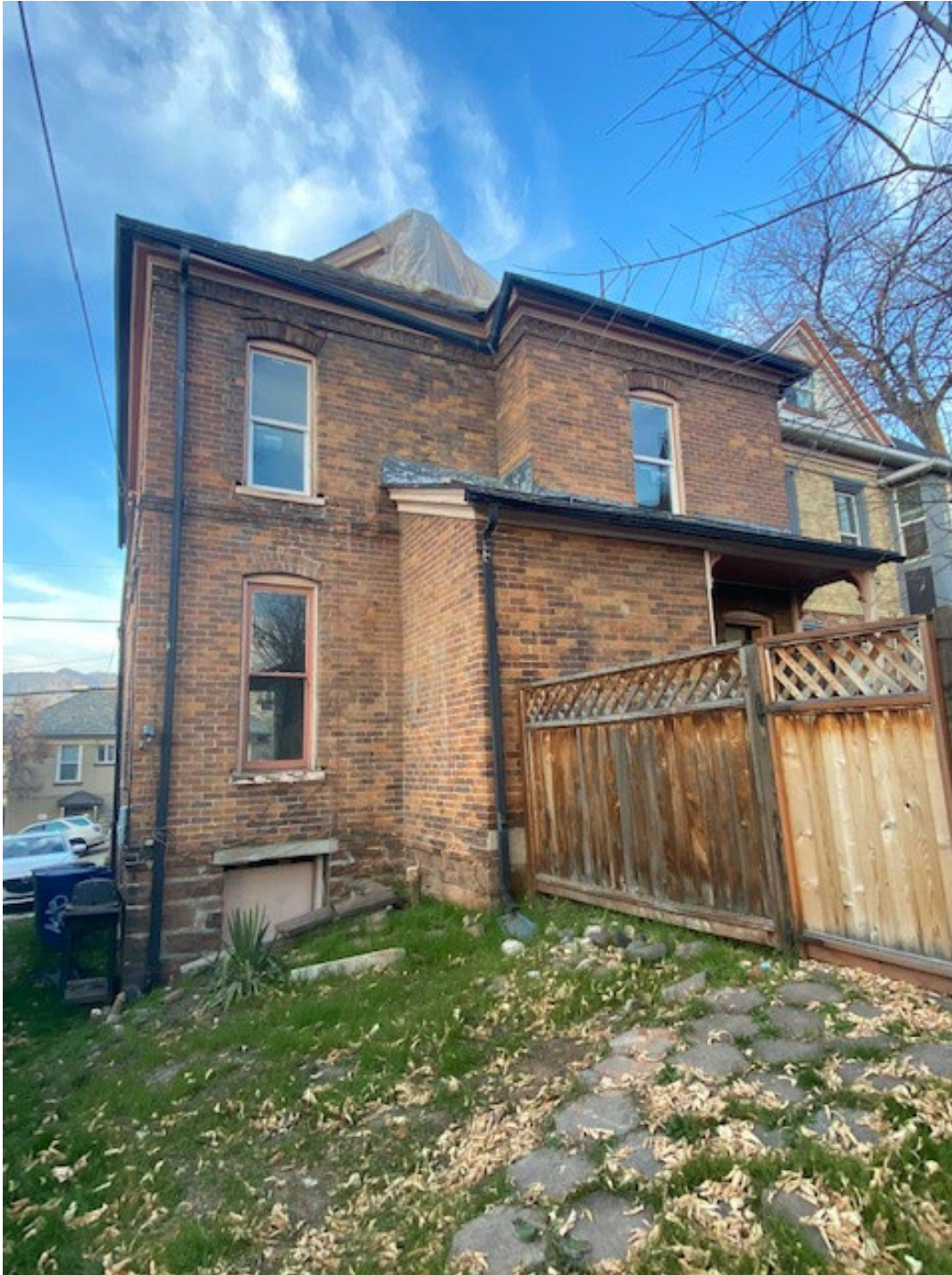
Figure 8: Photograph of rear (southern) facade provided by Applicant.
