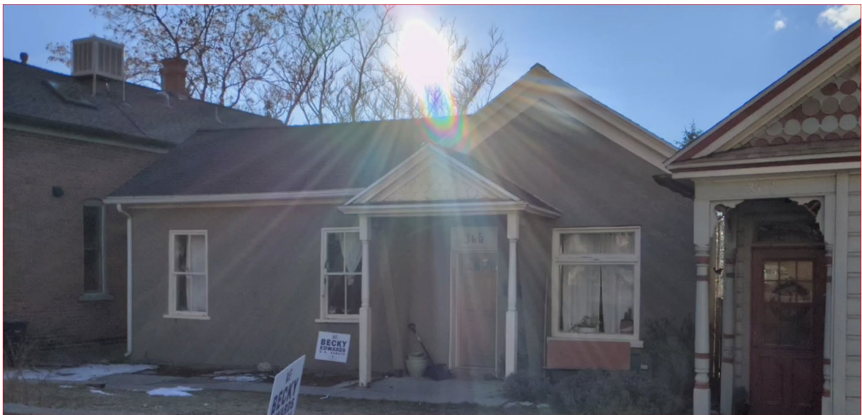
View of House, East Façade from Street
