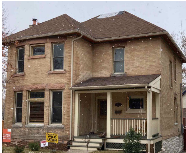
Image 5 – View of front façade 740 E 3 rd Ave.
