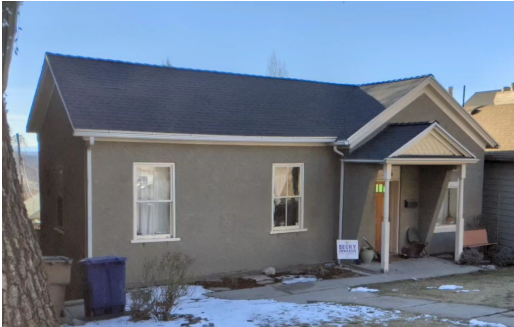
Image 1 – Front (east) façade of house. View of the roof pitch.
