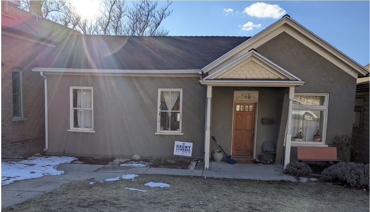
View of House, East Façade from Street
