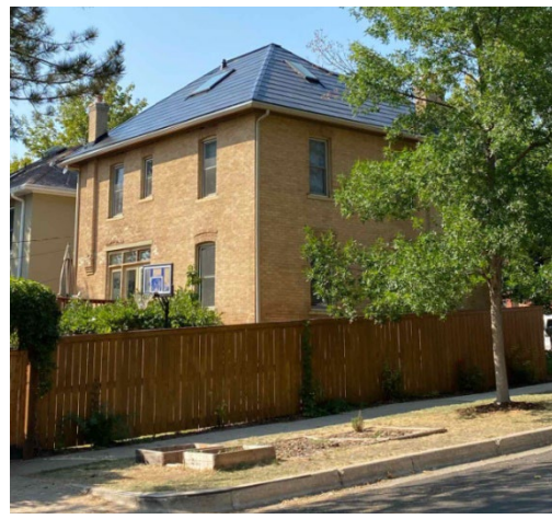
Image 4 – View of side and rear façades of completed installation.
