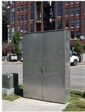
S12. Electrical Large Box
