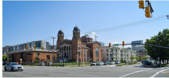
X2. Northeast End, 300 S & 300 W (Looking Northeast)
