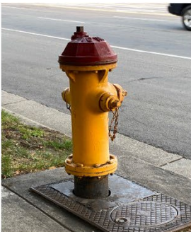
S29. Fire Hydrant
