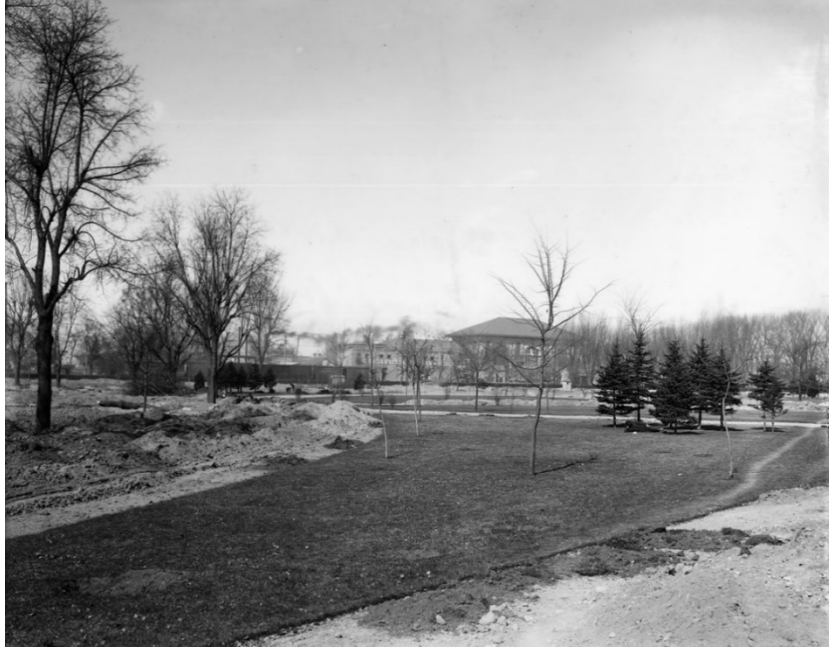
Figure 4.2.1: Late 1910 photo looking northwest across the park, with the Denver & Rio Grande Depot visible in the background. The piles of dirt visible in the foreground and on the left indicate that this image was taken mid-construction.
