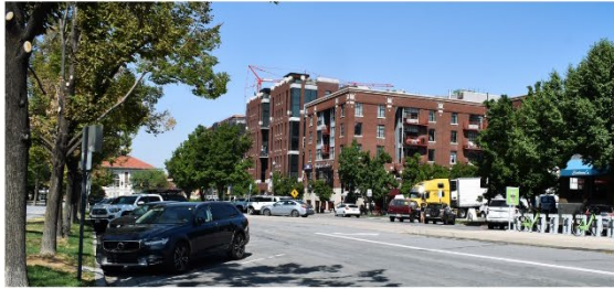
X1. North End, 300 South (Looking Northwest)
