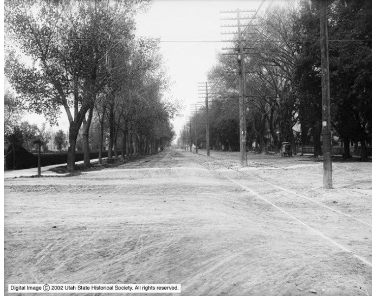
Figure 4.1.3: 1909 photo of street paving looking south along 400 West. Pioneer Park is visible on the left-hand side of the historic image. This photo illustrates the sidewalk, park strip and street tree configuration defining the perimeter of the park. A clipped hedge lined the inside of the public sidewalks. A portion of the corner entrance to the park is visible.
