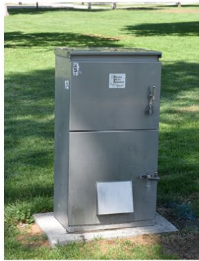
S11. Electrical Box
