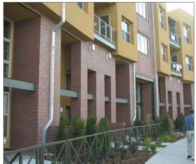
Deeply recessed windows and doors on lower floors create a strong sculptural base for the articulation of the facade above.
