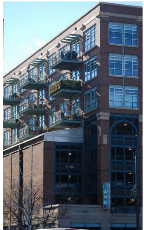
The window frame pattern and profiles effectively used to embellish facades and screen parking decks.
