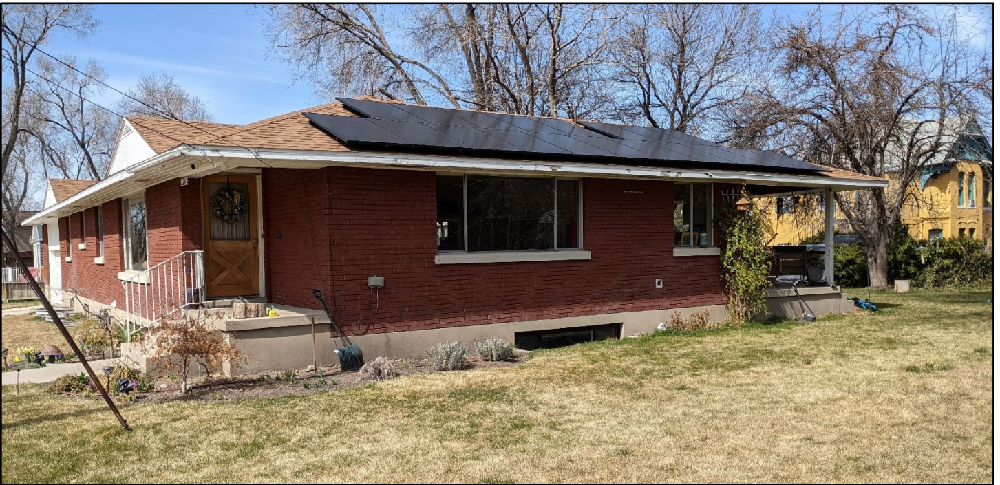
East façade of the subject property
