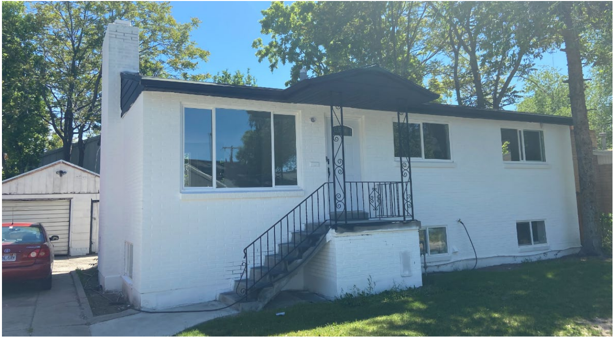
View of House After Paint Applied, South/West Perspective from Ardmore Place
