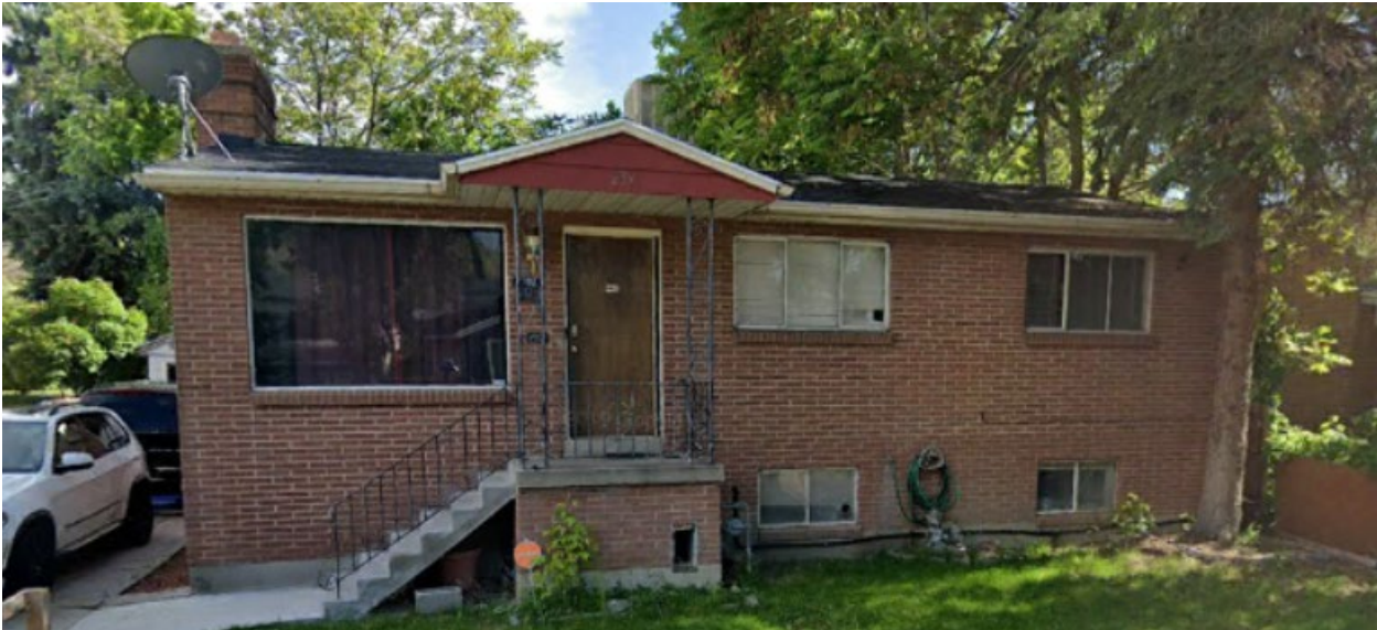
Image 1 – Front (north) façade of the apartment building before paint work was completed.
