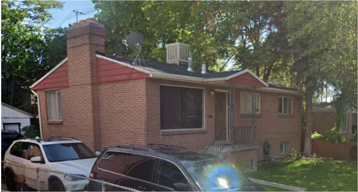
View of House Before Brick was Painted, from Ardmore Place South/West Perspective
