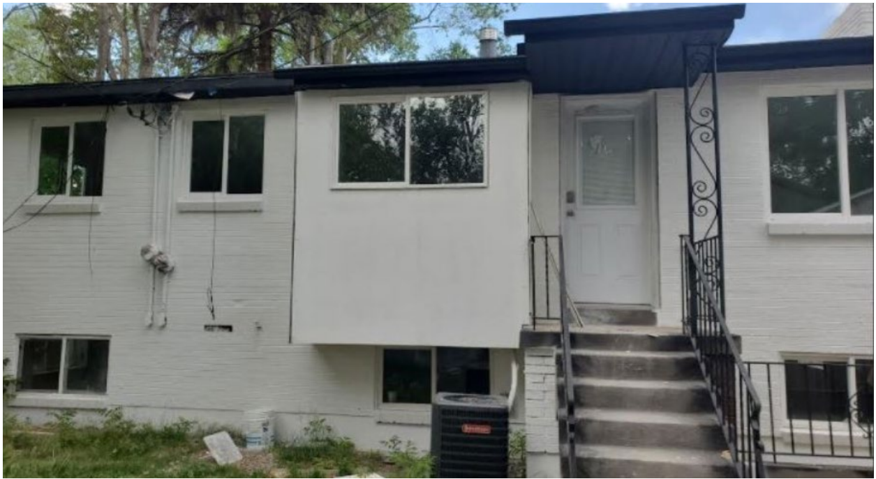
View of House After Paint Applied, Rear Facade
