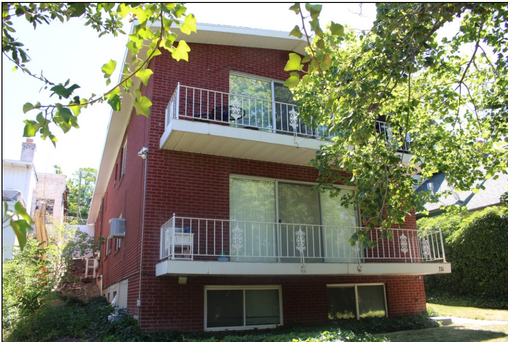
Photograph 7 of 10: Example of Ranch form dwelling; 331 S. 1100 E.; camera facing east
