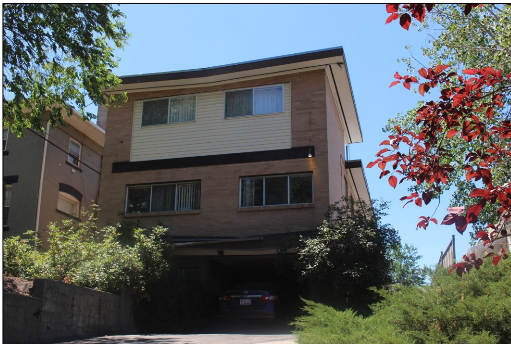
Photograph 5 of 10: Example of duplex from extended period of significance; 1154 E. 300 S.; camera facing southeast
