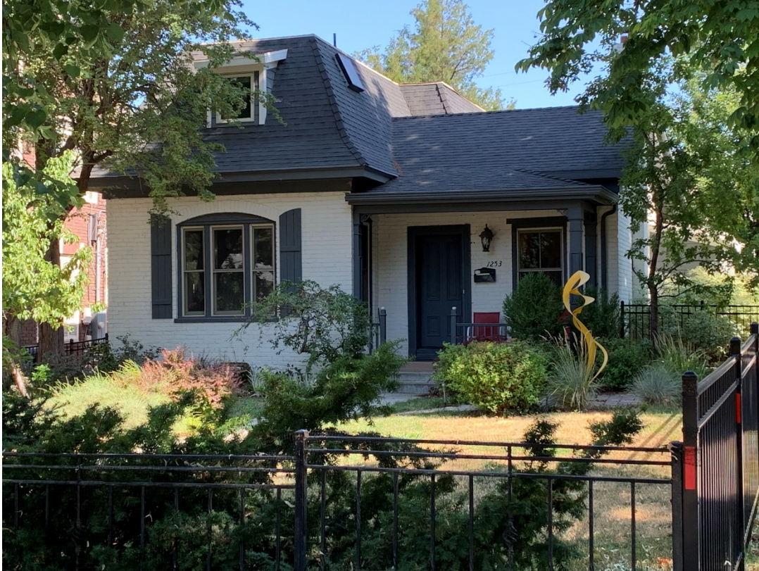
Image 1 – Front (south) façade of the building after paint work was completed.
