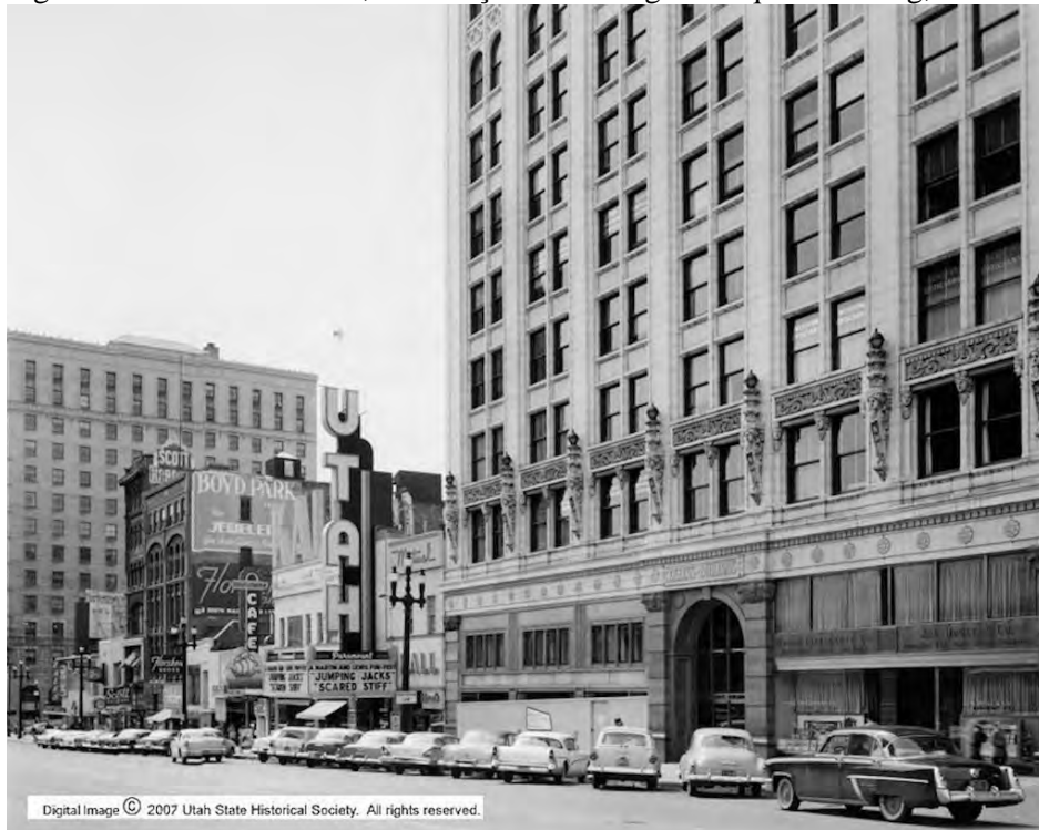
Figure 14. Historic exterior, main façade with larger marquee lettering, view southwest, 1958.
