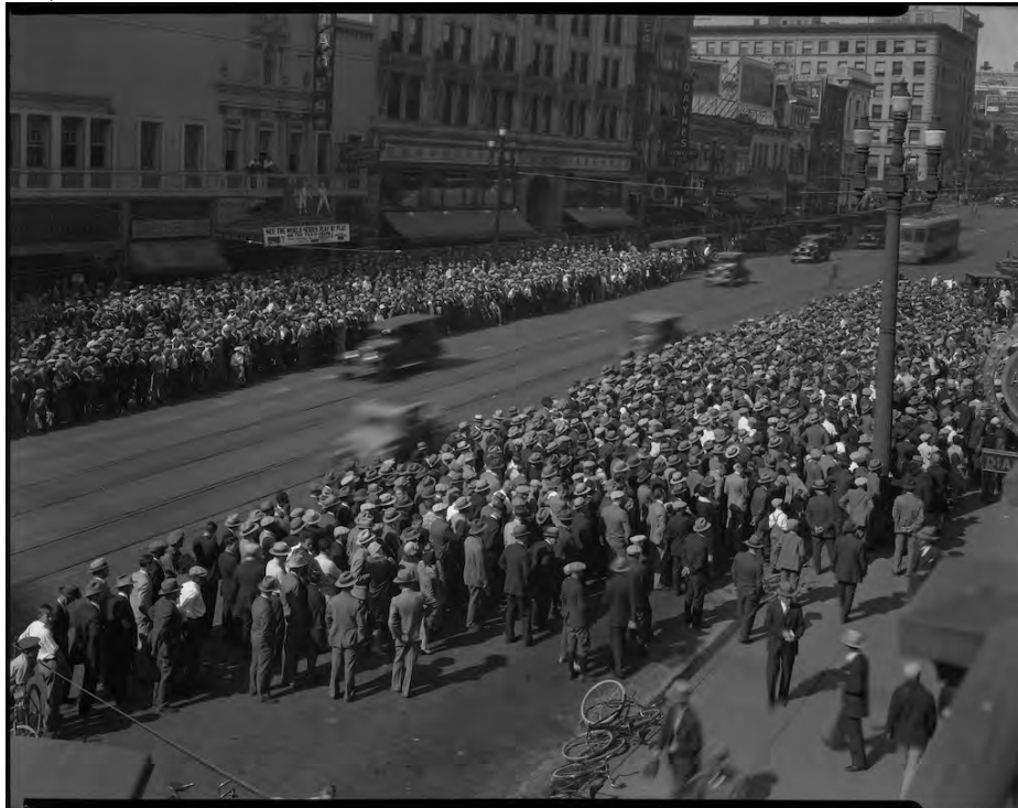
Figure 10. Historic exterior, crowd watching the World Series in front of and at the Pantages Theatre (top left), view northwest, 1928.
