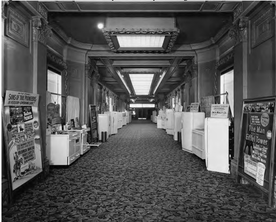
Figure 13. Historic interior, Entry Hall/Lobby showing modernization, view west, 1950.
