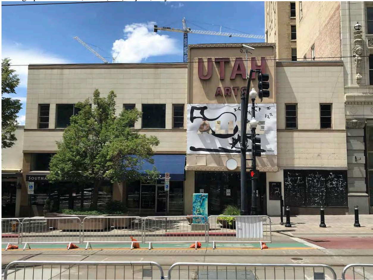
Photograph 1. Exterior, main (east) façade, July 2021. Camera view west.
