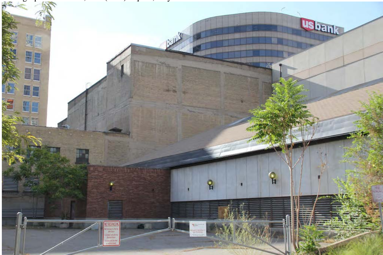
Photograph 4. Exterior, rear (west) façade, July 2021. Camera view southeast.
