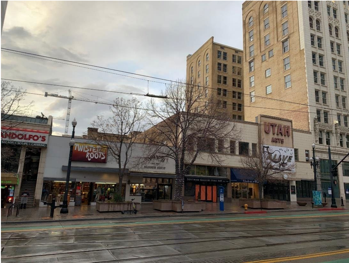
Pantages/Utah Theater Building, 2021
