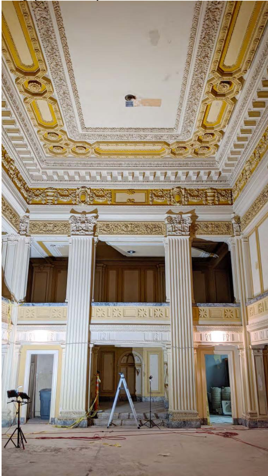
Photograph 8. Interior, Foyer, October 2020. Camera view north.
