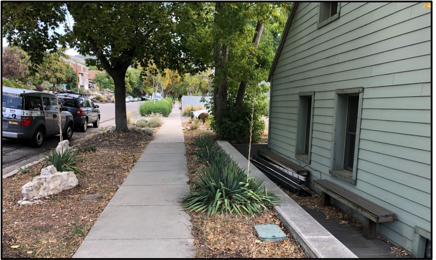
View of Sidewalk in front of subject property looking east
