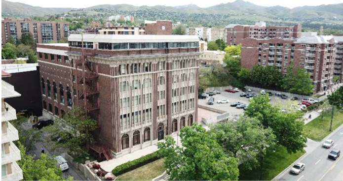
Existing Elks Building and Site
