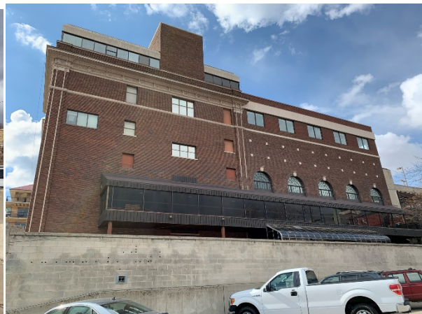
Figure 1 - East Side with existing roof addition, greenhouse and filled window openings. The stair/elevator tower will also be relocated to the center of the building.
