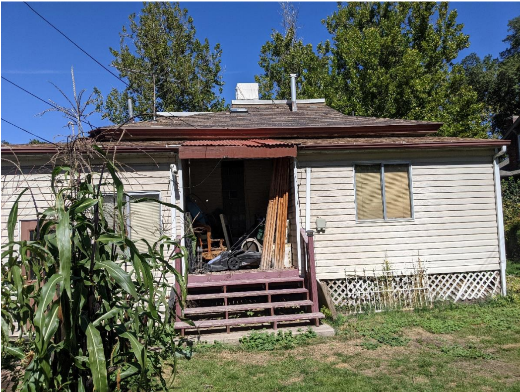
Rear/South façade, showing rear addition and covered porch
