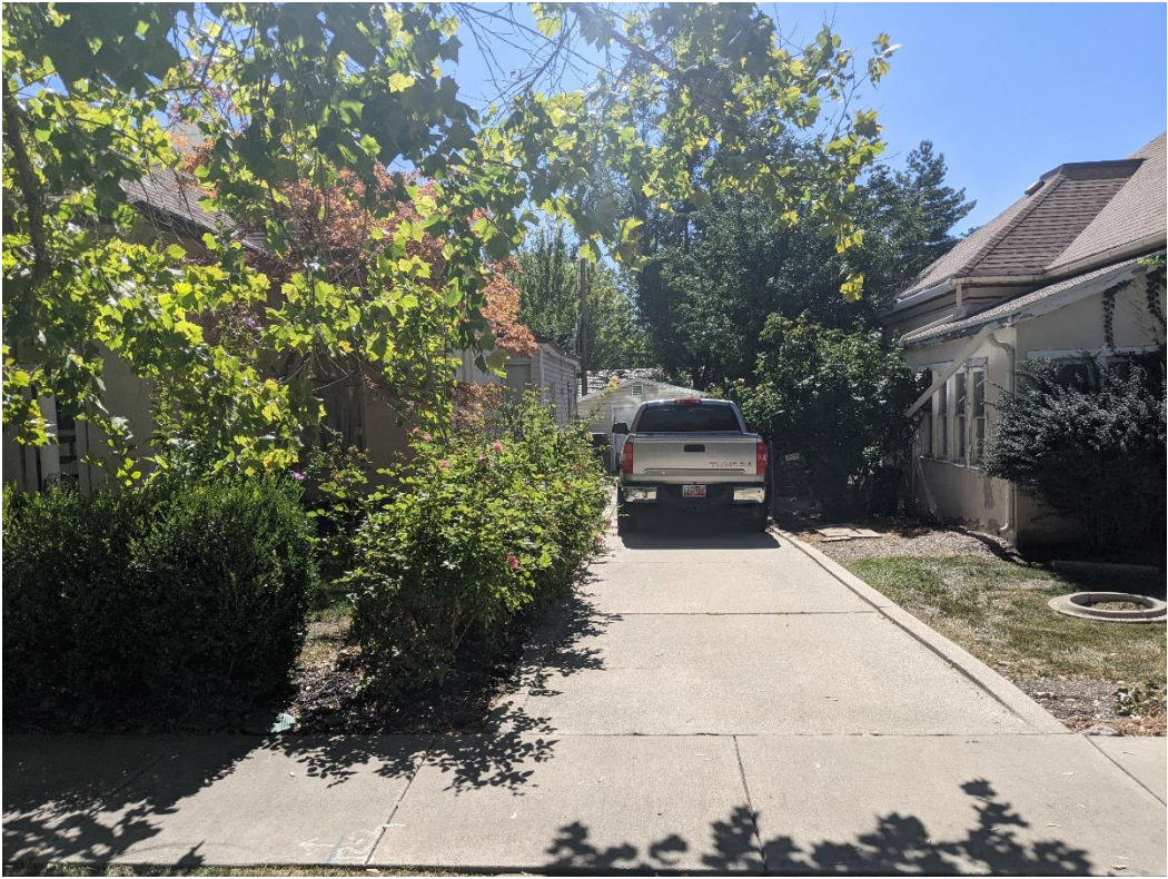
View of detached garage from 2 nd Avenue
