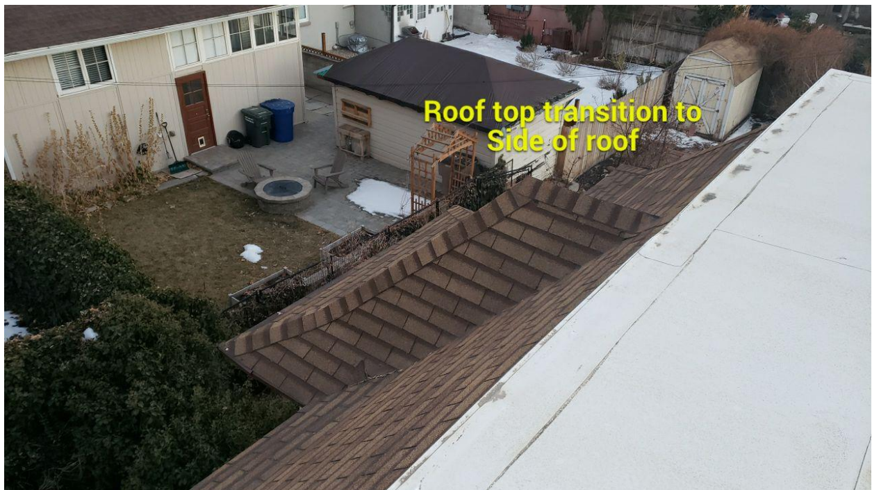
Materials showing sections of roof proposed to be replaced
