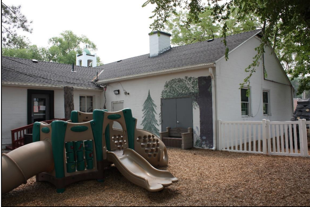
Photo 19 of 54. North and west elevations of the west addition to the Mexican Branch meetinghouse. Camera facing southeast.
