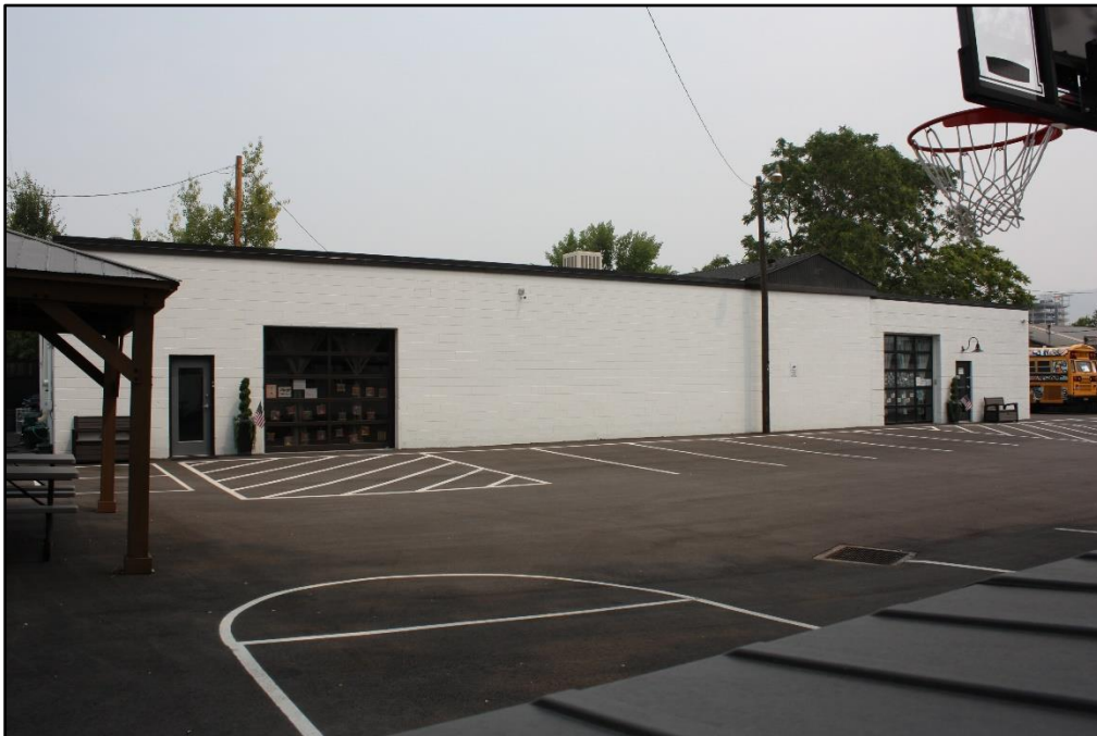
Photo 53 of 54. South elevation of the non-contributing building behind (north of) the Mexican Branch meetinghouse. Camera facing northeast.
