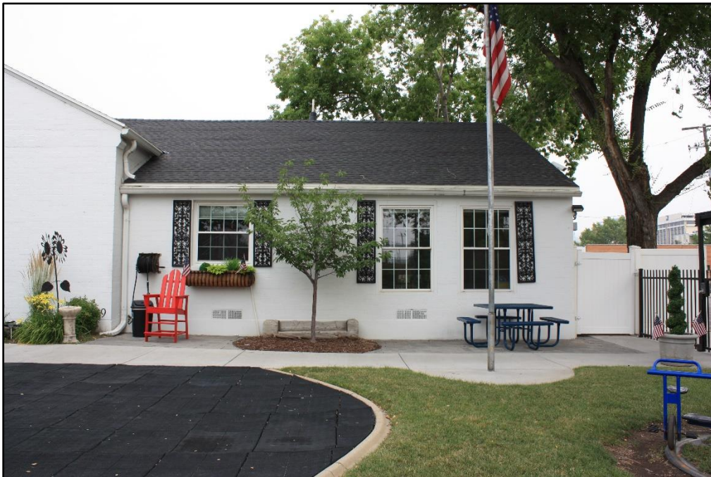
Photo 10 of 54. East addition to the Mexican Branch meetinghouse, Bays A and H of the south elevation. Camera facing north.
