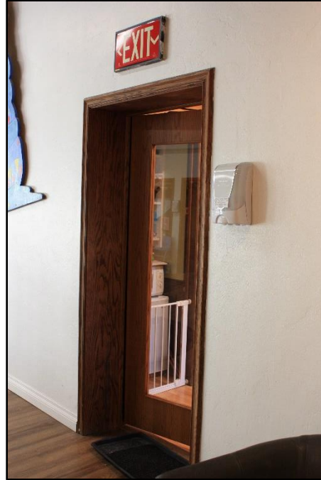
Photo 27 of 54. Entrance to the east addition in the original concrete block wall of the east elevation of the Mexican Branch meetinghouse. Camera facing northeast.
