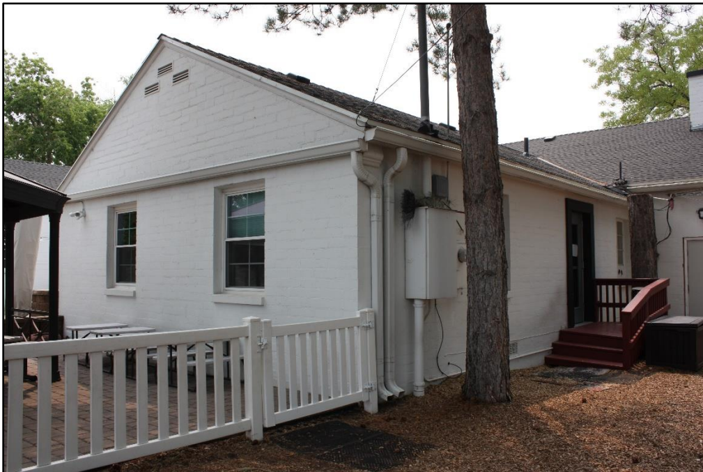
Photo 18 of 54. North and west elevations of the west wing of the Mexican Branch meetinghouse. Camera facing southeast.
