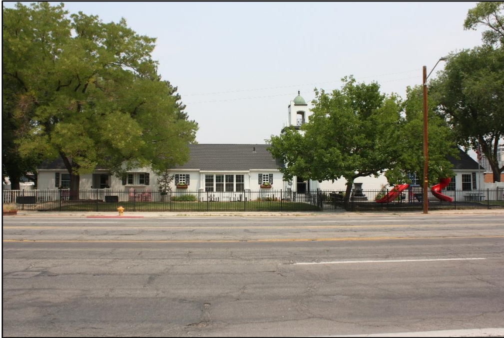
Photo 1 of 54. Overview of the Mexican Branch meetinghouse south (primary) elevation. Camera facing north.
