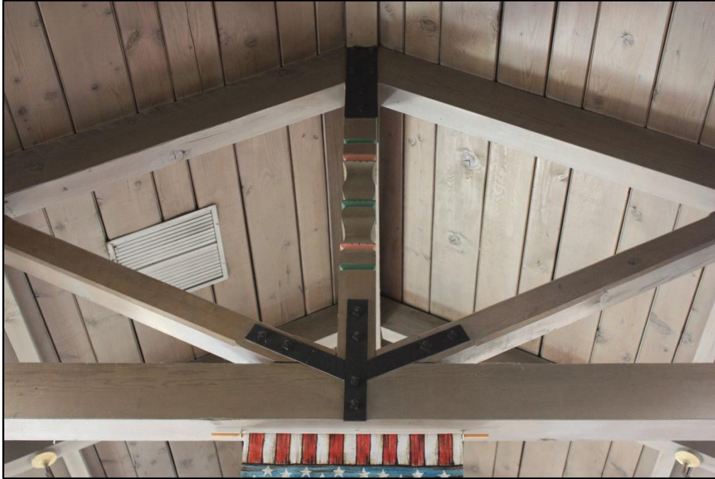
Photo 25 of 54. Detail of truss and wood ceiling in the chapel of the Mexican Branch meetinghouse.
