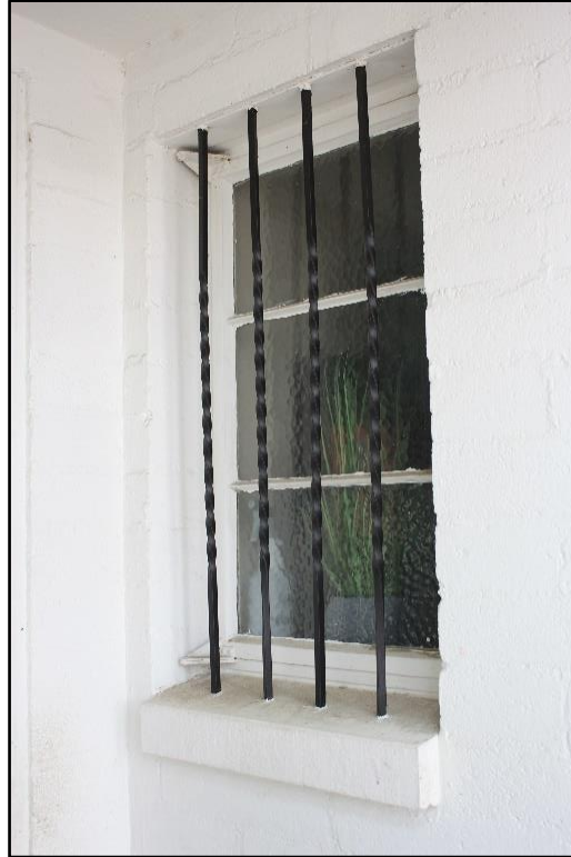
Photo 5. Detail of the original window in west elevation of branch president's office of the Mexican Branch meetinghouse. Camera facing north.
