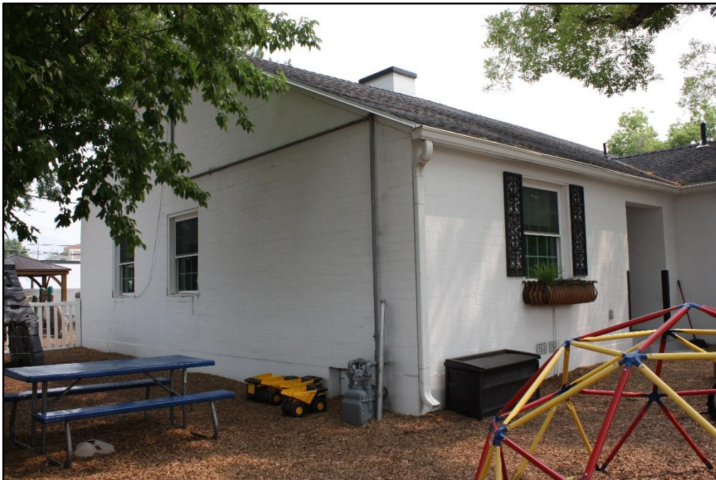
Photo 20 of 54. West and north elevations of the west addition to the Mexican Branch meetinghouse. Camera facing northeast.
