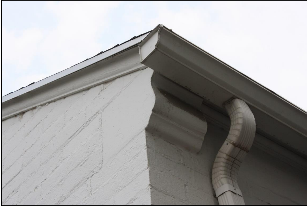
Photo 9 of 54. Detail of curvilinear quoin bracket at the southeast corner of the east wing. Camera facing northwest.
