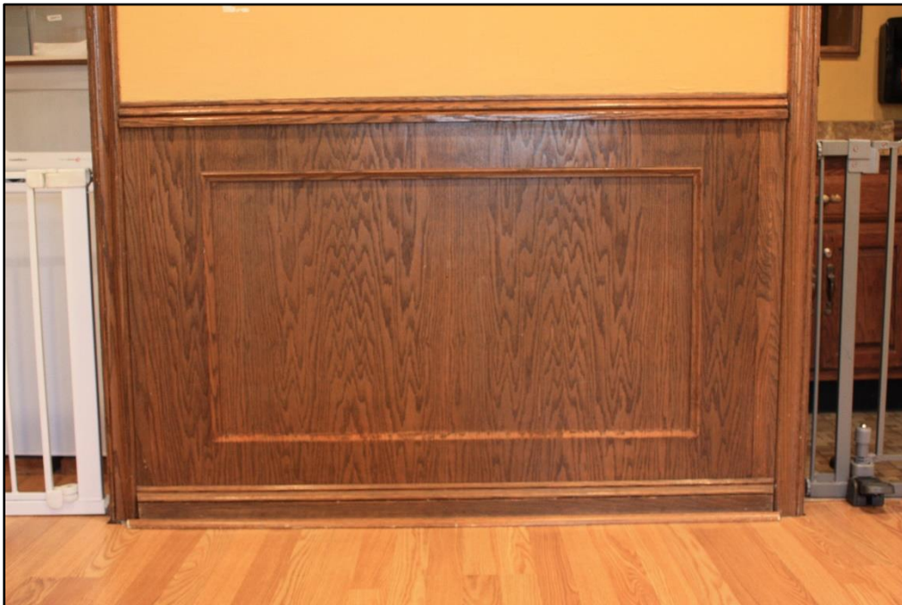
Photo 30 of 54. Detail of original wood wainscoting in the east addition of the Mexican Branch meetinghouse.
