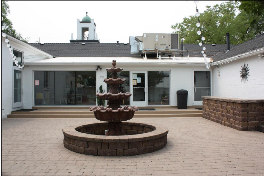
Photo 17 of 54. North elevation of the recreation/cultural hall of the Mexican Branch meetinghouse. Camera facing south.
