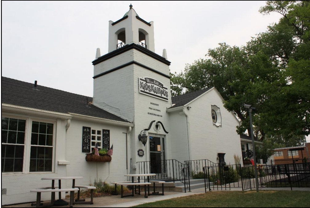
Photo 7 of 54. Original Mexican Branch meetinghouse entrance, Bays F and G of the south elevation. Camera facing northeast.
