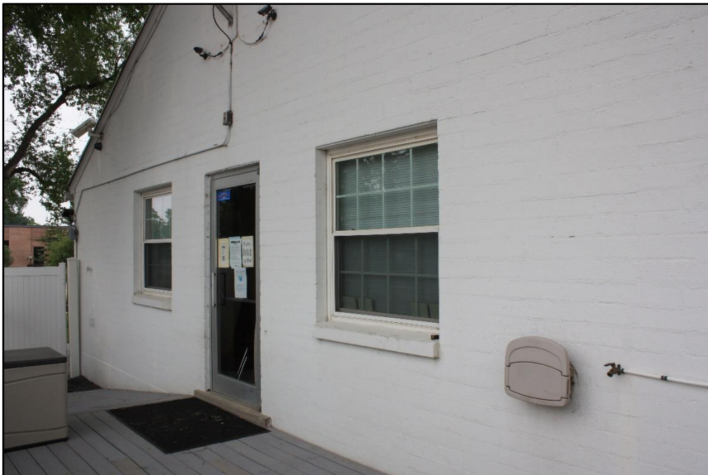
Photo 12 of 54. East elevation of the east addition, Bays A, B, and A. Camera facing southwest.
