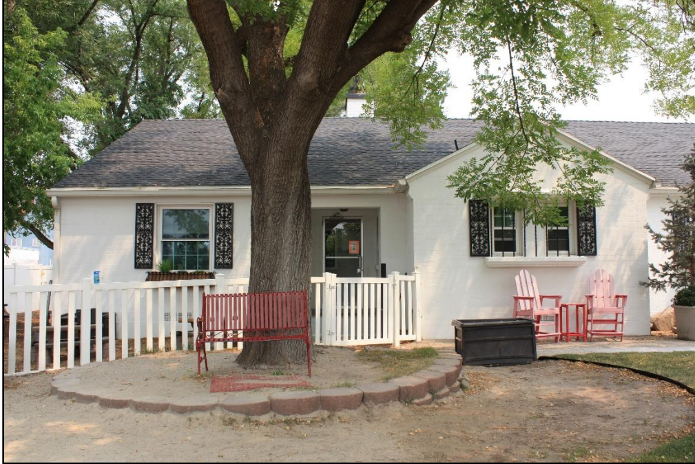
Photo 3 of 54. West addition (left) and the original Mexican Branch meetinghouse, Bays A, B, and C of the south elevation. Camera facing north.
