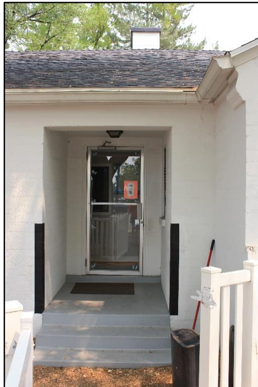
Photo 4 of 54. Entrance into the west addition with typical aluminum glazed door. Camera facing north.
