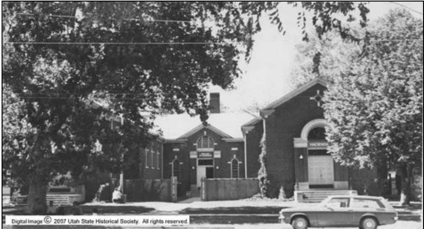
Figure 40. “Catholic Church, Our Lady of Guadalupe. The Hacienda (right) served as a place for community services for Spanish speaking people of Salt Lake City.” 1976. The building, formerly at 129 North 600 West, has since been demolished. (Utah State Historical Society Classified Photograph Collection, Photograph No. 08169, courtesy of Utah State Historical Society).
