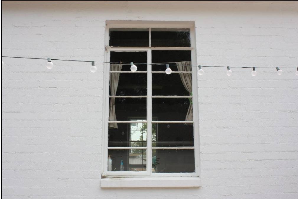
Photo 15 of 54. Detail of original two-by-four casement window with transom in the west elevation of the chapel in the east wing of the Mexican Branch meetinghouse. Camera facing east.
