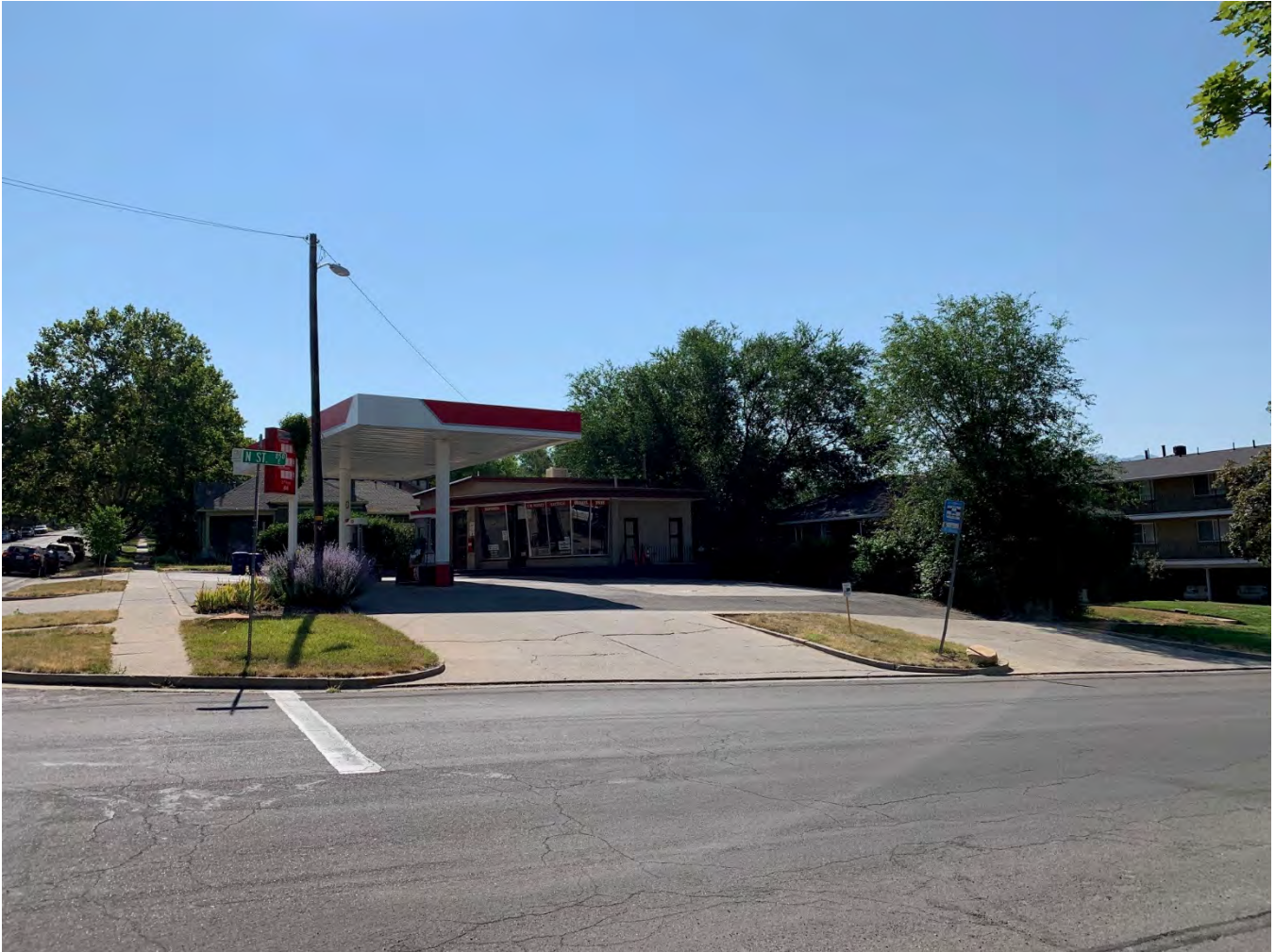
Figure 10: View of existing service station as viewed from N Street.
