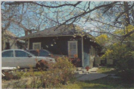
1007 E 1 st Avenue (garage)
