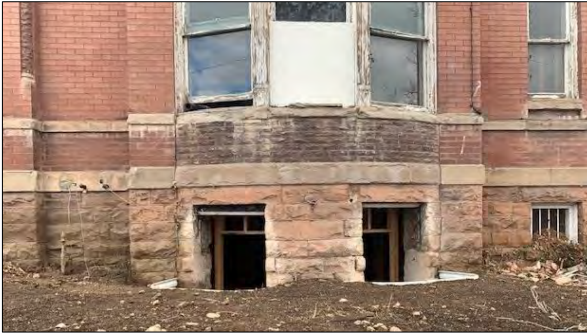
Post Enforcement Photo of West Elevation
