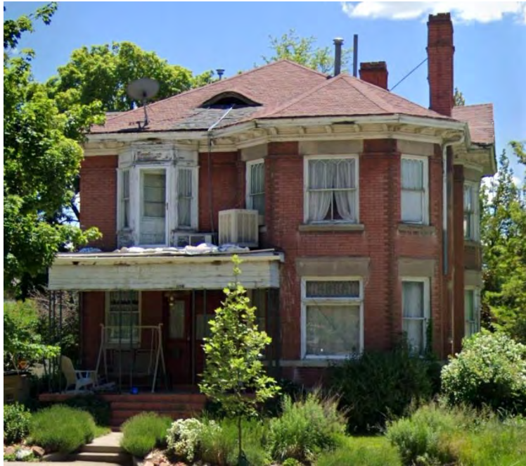
2019 Photograph of the Existing Porch
