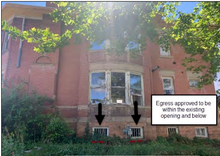
Photo of West Elevation
