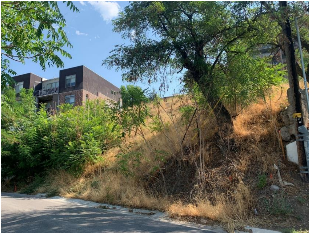
Existing Conditions – N. West Temple facing east
