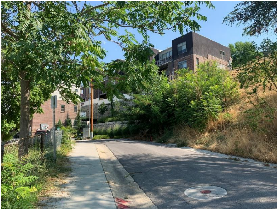
Rear of residence to the north and subject property from N. West Temple
