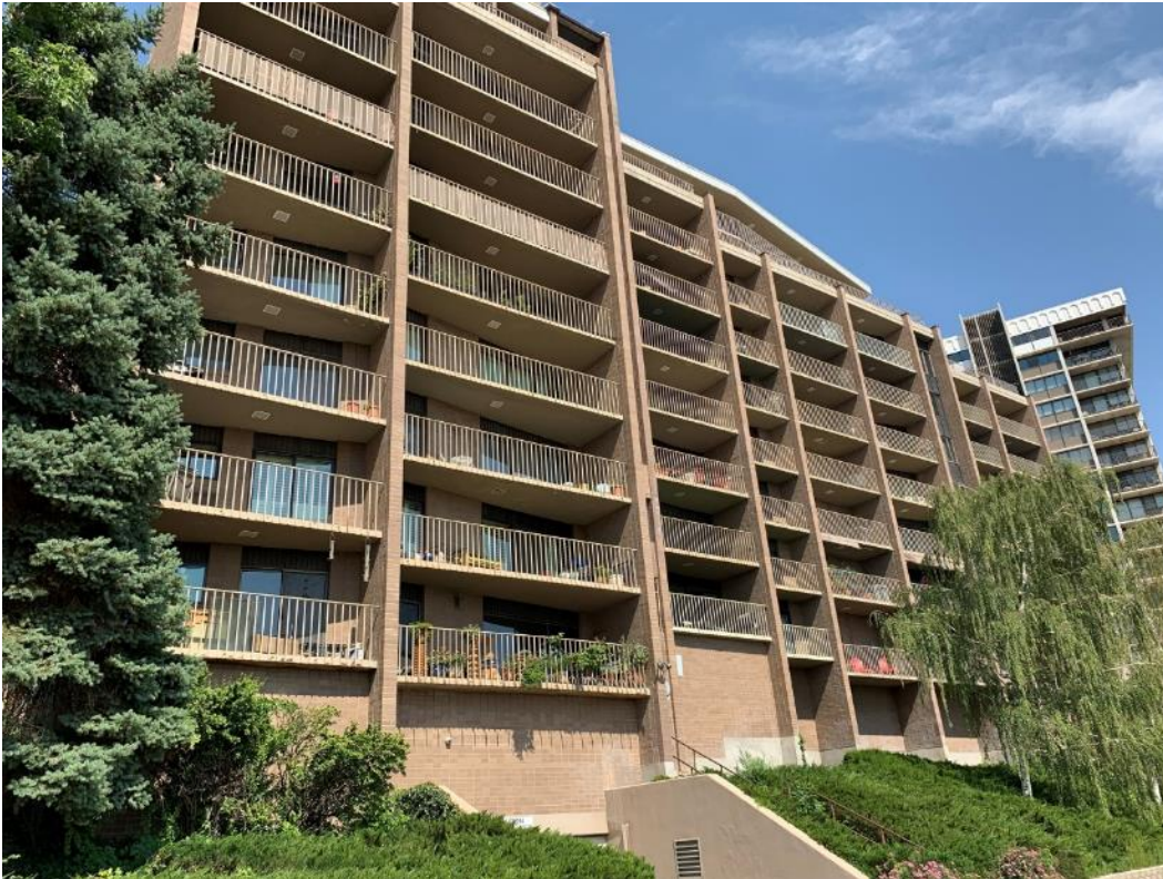
Rear of Trevi Towers, located southeast of the subject property.
