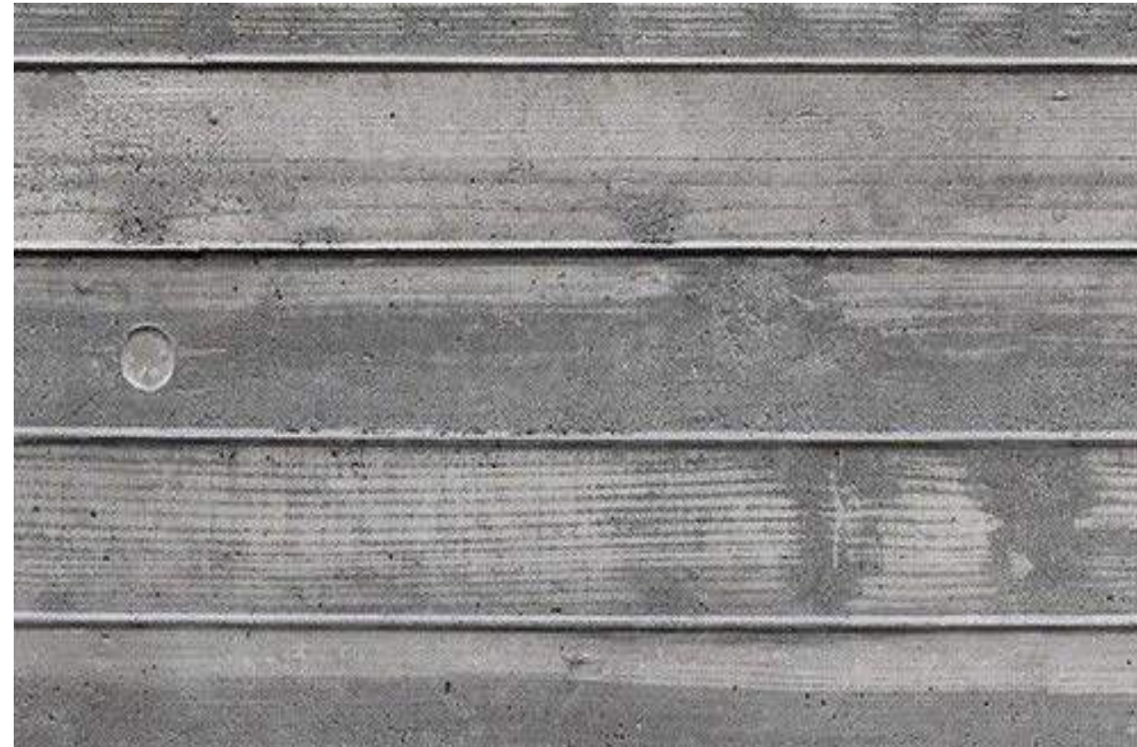
BOARD-FORM CEMENT DETAIL
