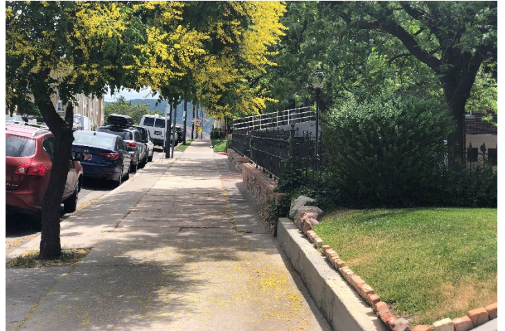
Existing fence from 1 st Ave looking east from sidewalk
