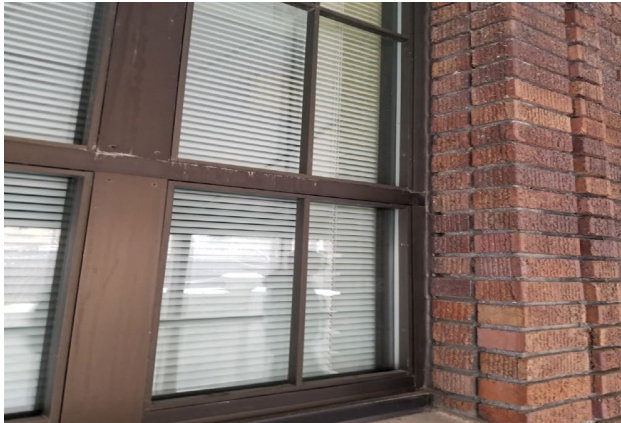
Figure 13 - Detail of window that has clearly been replaced.
