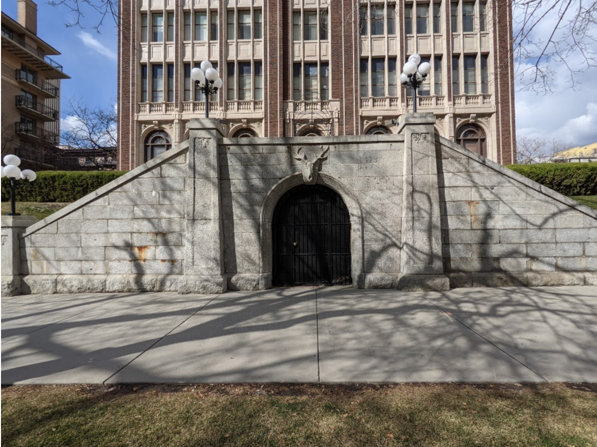
Figure 9 – Current tunnel building entry and stairs to main entrance.
