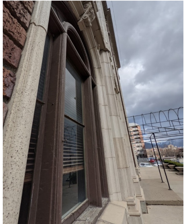
Figure 15 - Detail of first floor arched windows on front facade.
