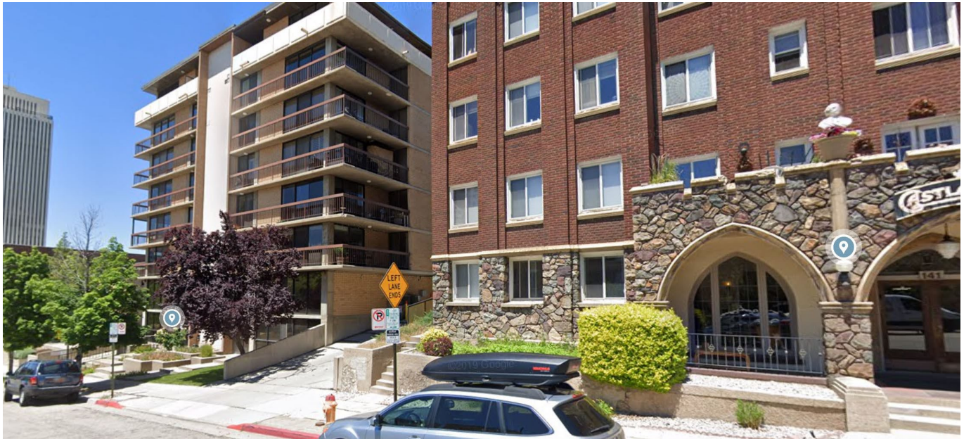
Surrounding development – North side of 1 st Avenue
