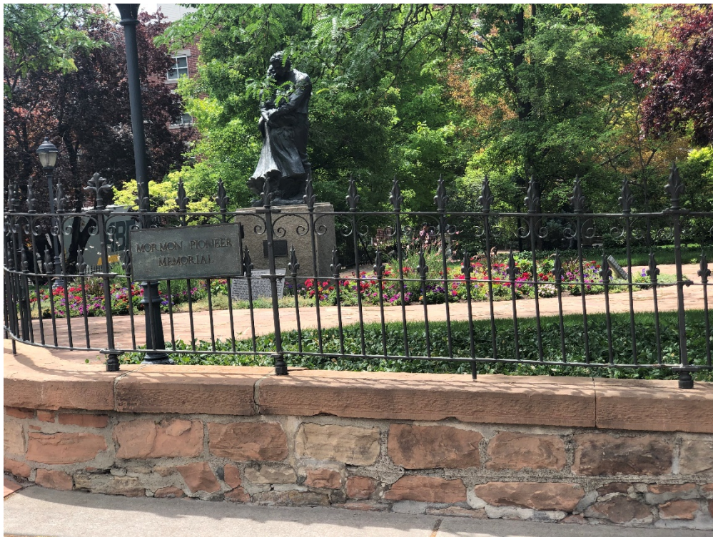
Existing fence along 1 st Avenue. The retaining wall and proposed fence will have a height of approximately 7 FT at the front property line along 1 st Avenue.
