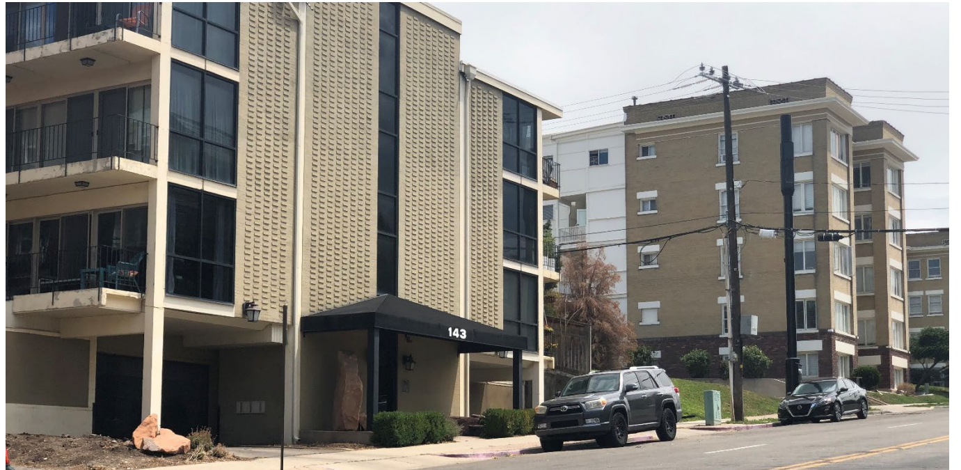
Surrounding development – North side of 1 st Avenue
