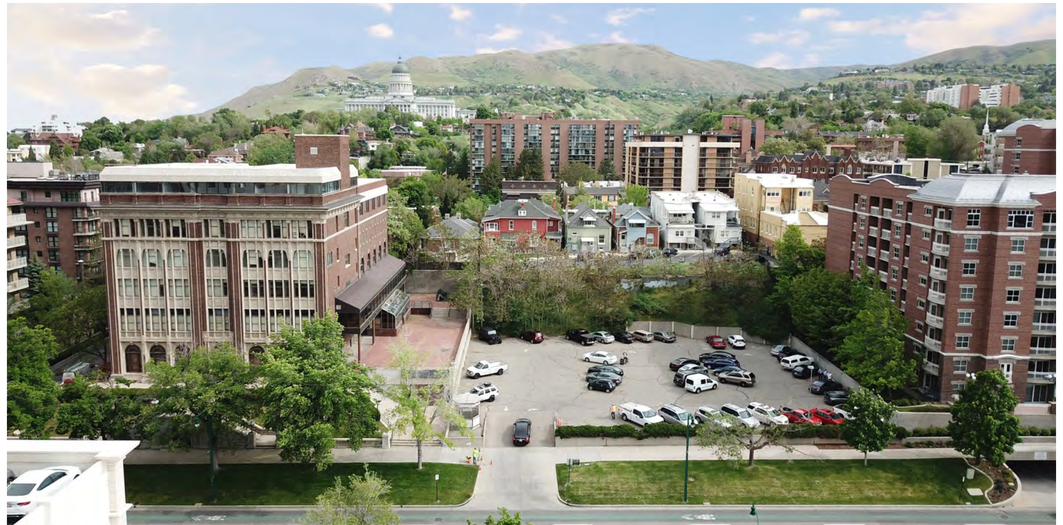
Existing Site Condition
