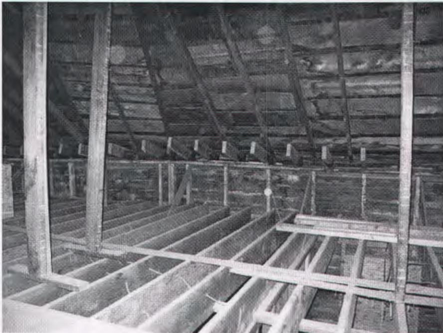
These 2x4's are the primary means of support for the roof structure.
