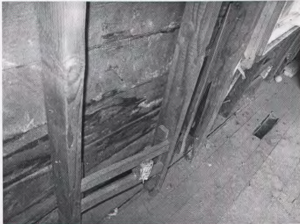
Examples of structural deficiencies.
