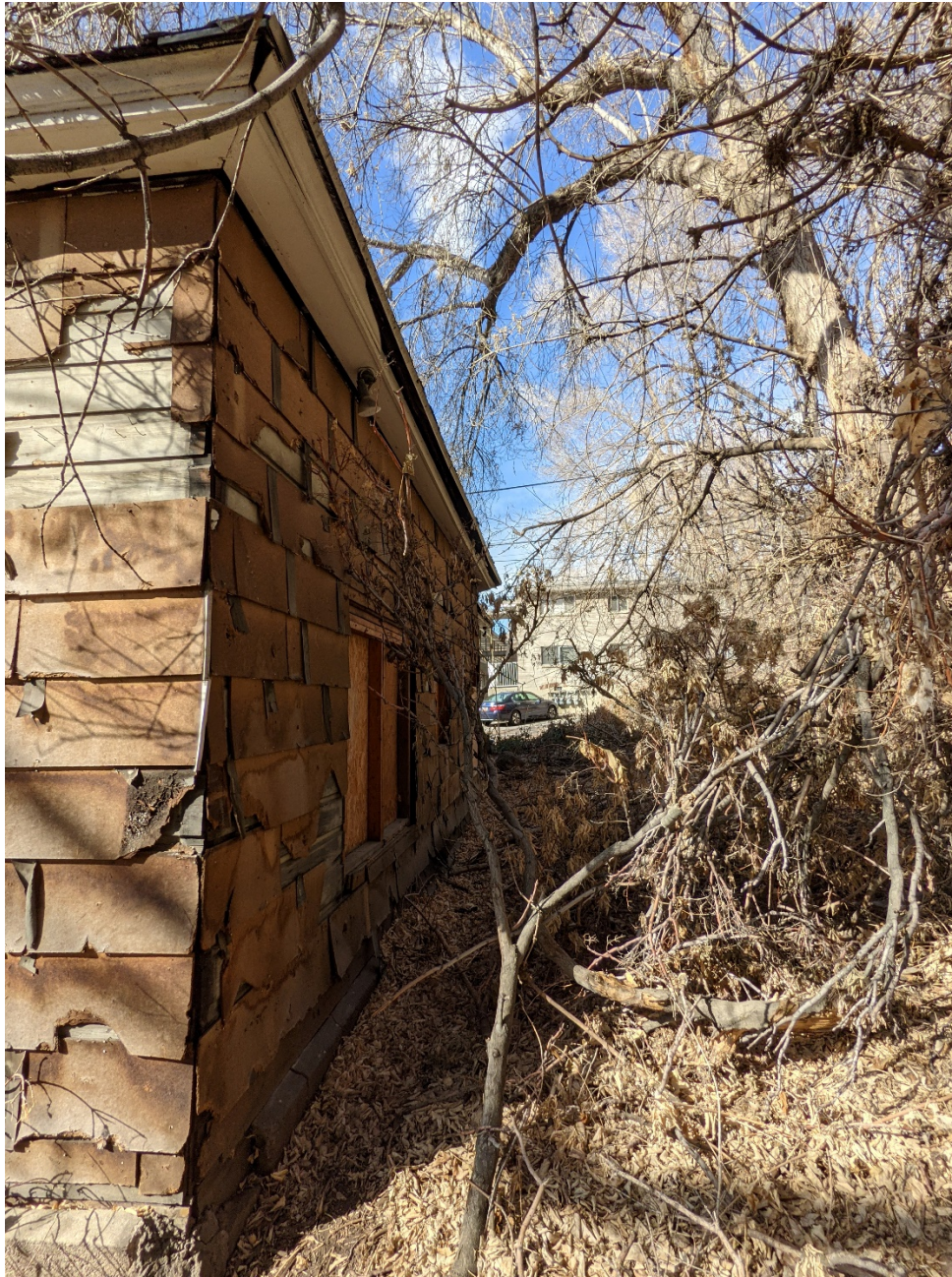
East Facade of Existing House – Looking North
