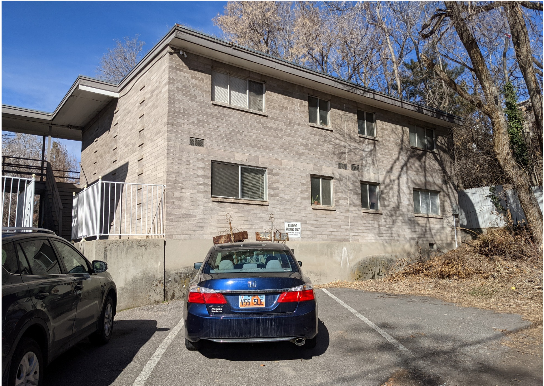
Rockcrest Apartments – Thistle Avenue Facade – Looking Northeast
