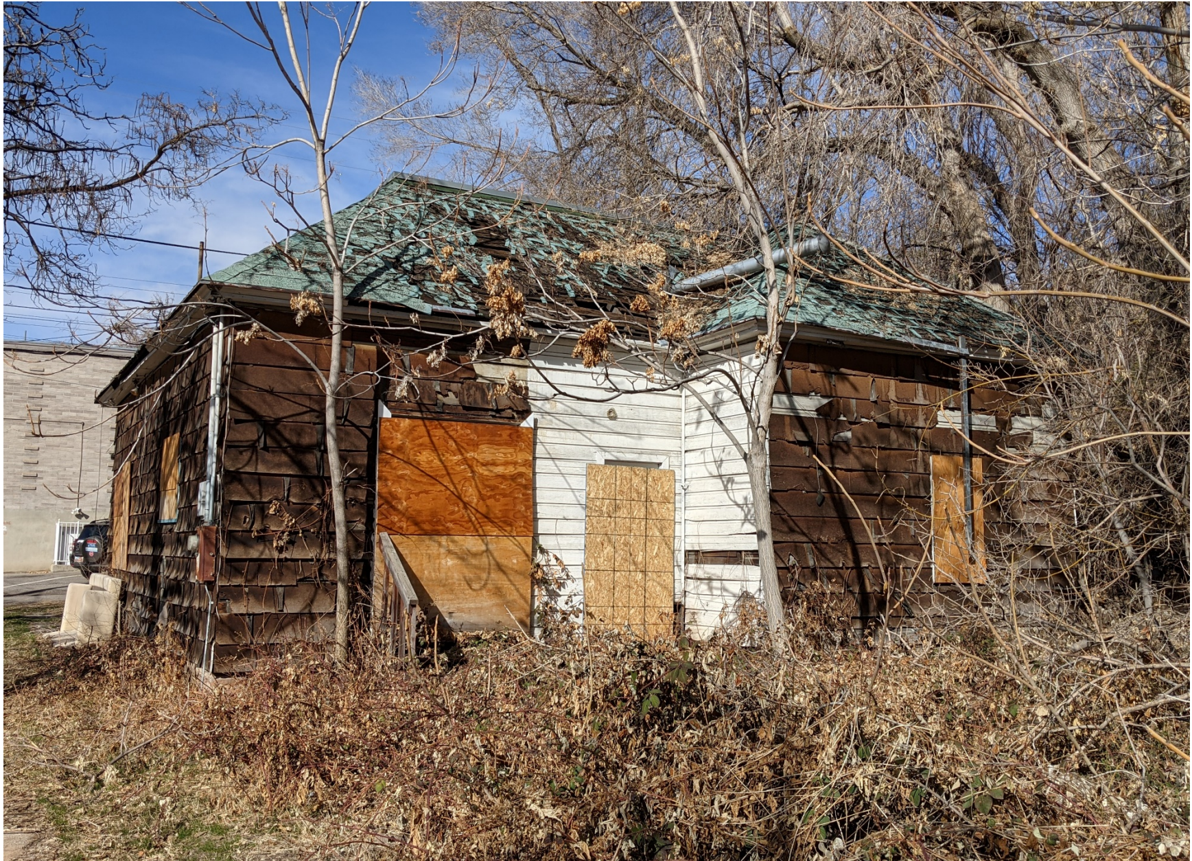
Existing House – Rear Facade – Looking North
