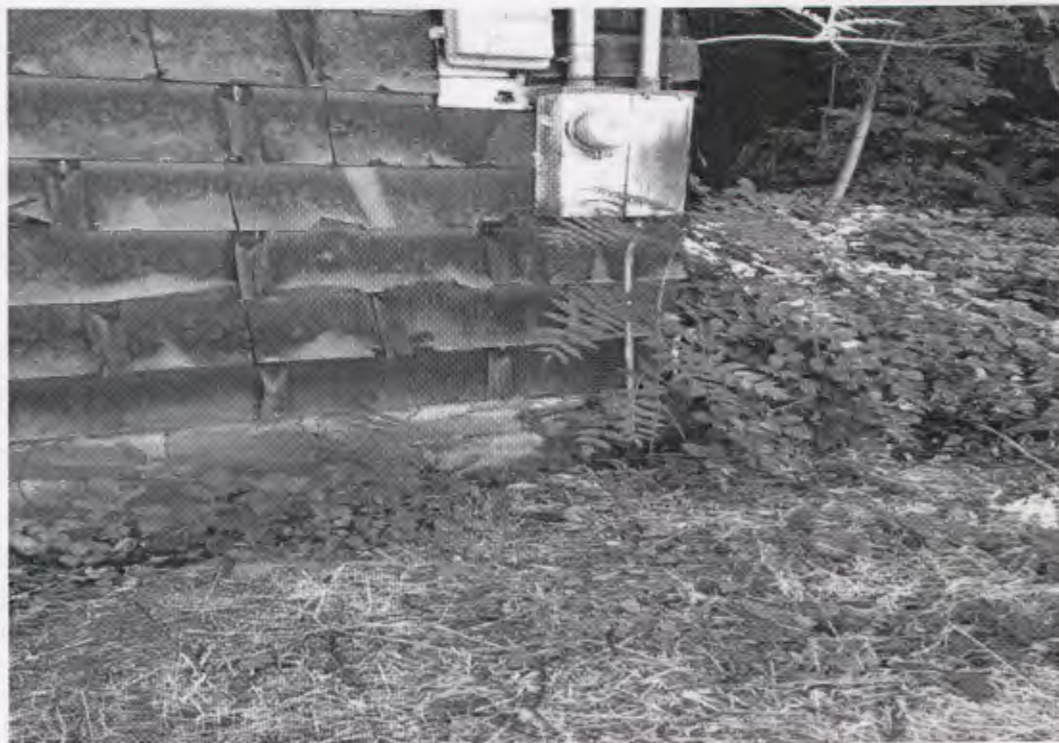
Photo 2: Stone and mortar foundation walls
