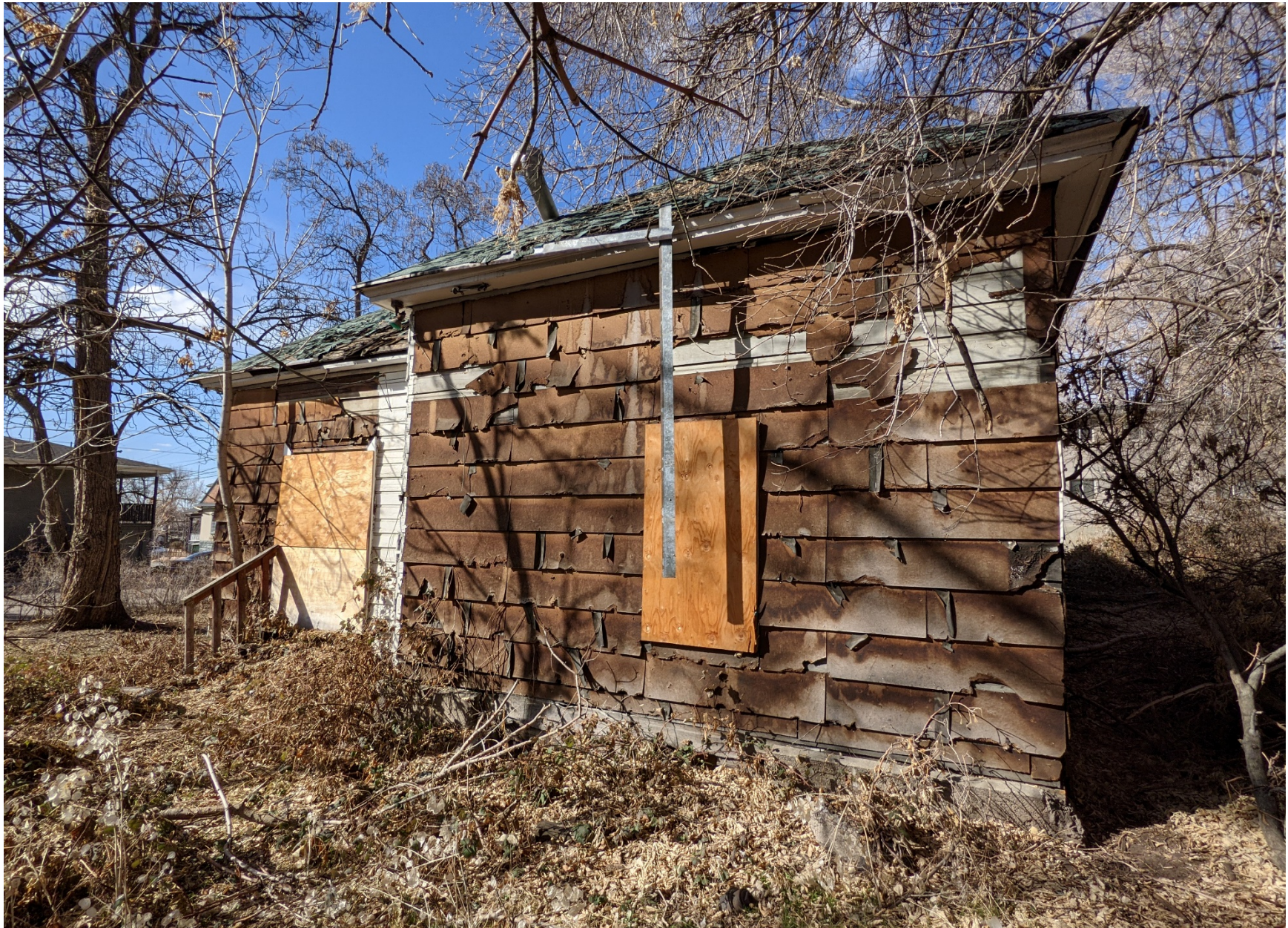
Rear of Existing House – Looking Northwest
