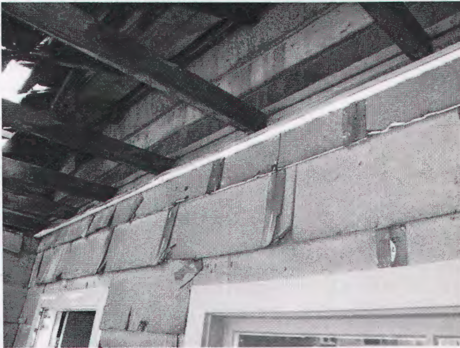
The porch itself has been removed and replaced. Current porch has been toenailed into siding.
