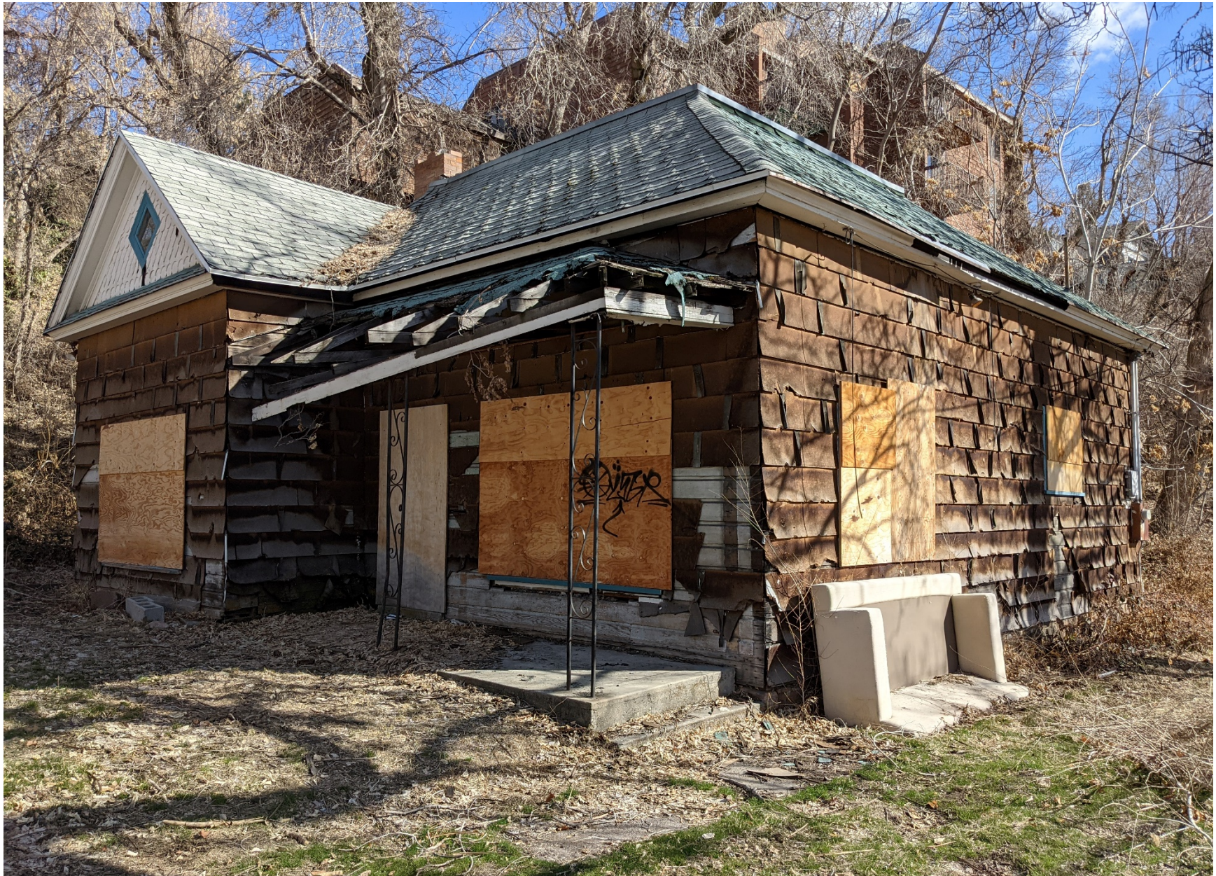
Existing House – Northwest Corner – Looking Southeast
