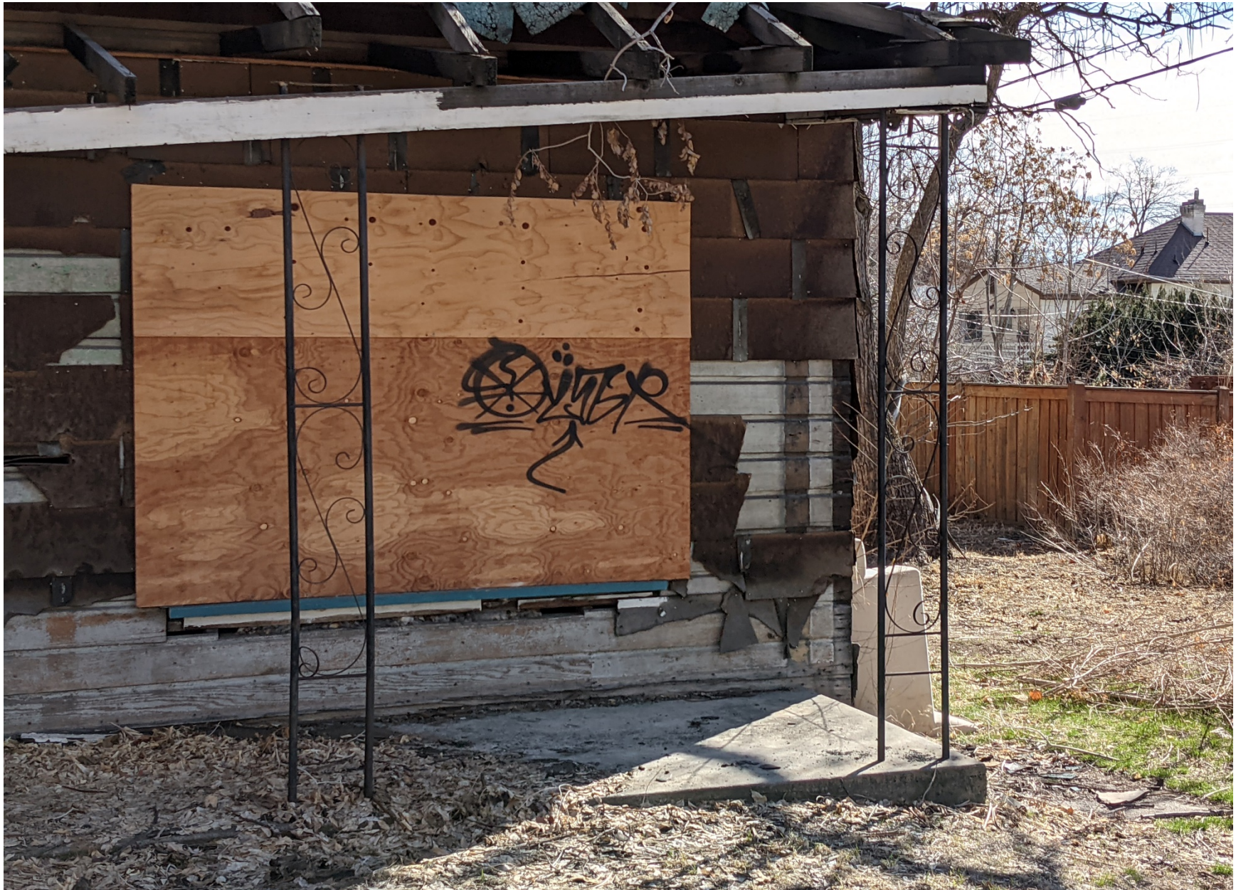
Existing House – Porch Detail
