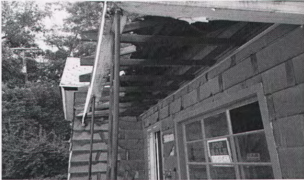
Photo 11: Deteriorated front porch beam
