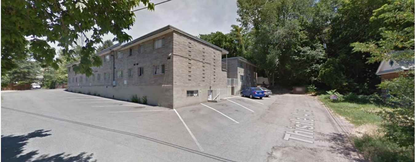
North Side of Thistle Avenue showing Rockcrest Apartments
