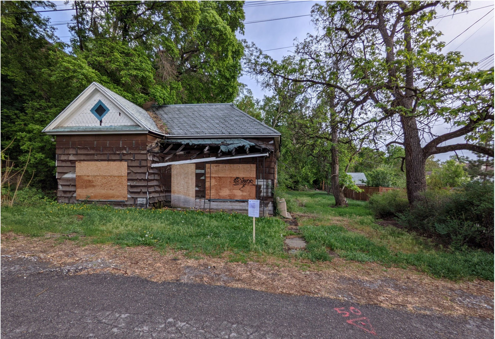
View of Existing Site – Looking South
