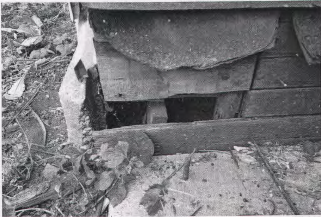
Photo 8: Deteriorated framing
