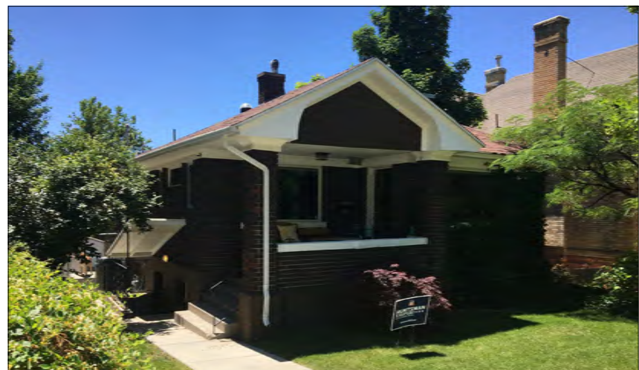
K1 Third Avenue Street View - Existing G0.2 1/4" = 1'-0"
