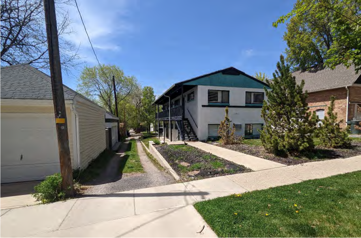
View of parallel alley from S Street – Looking south toward R Street
