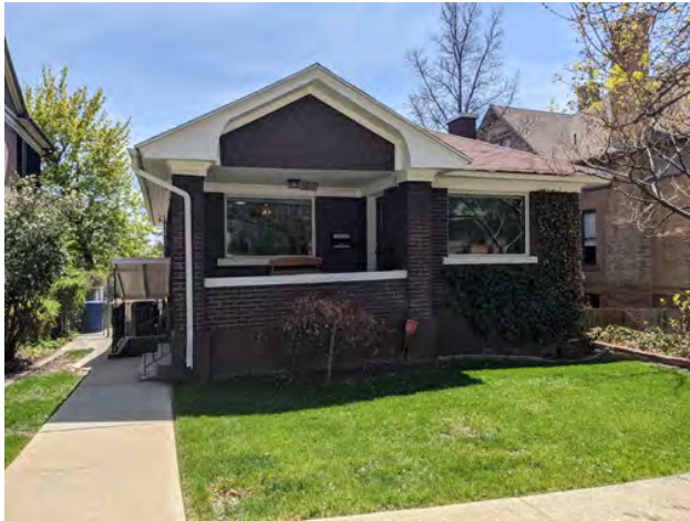
Existing house at 1076 E 3 rd Avenue, built in 1925 for the Leon F. Browning Family.
