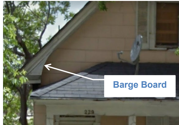
Front façade gable showing aluminum fascia and before the barge board was removed.
