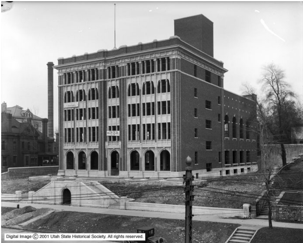
Elks Building Under Construction – 5 December 1922
