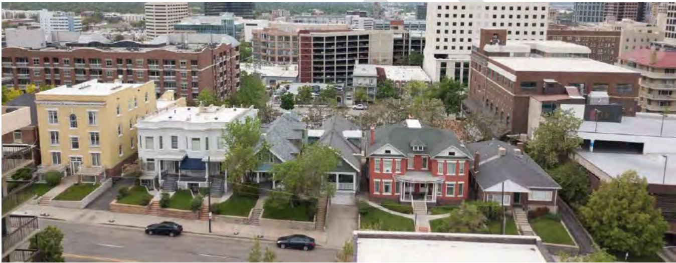
Existing Site from N looking S 1 st Avenue Streetscape
