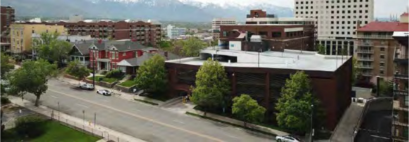
Existing Site from NW looking SE
