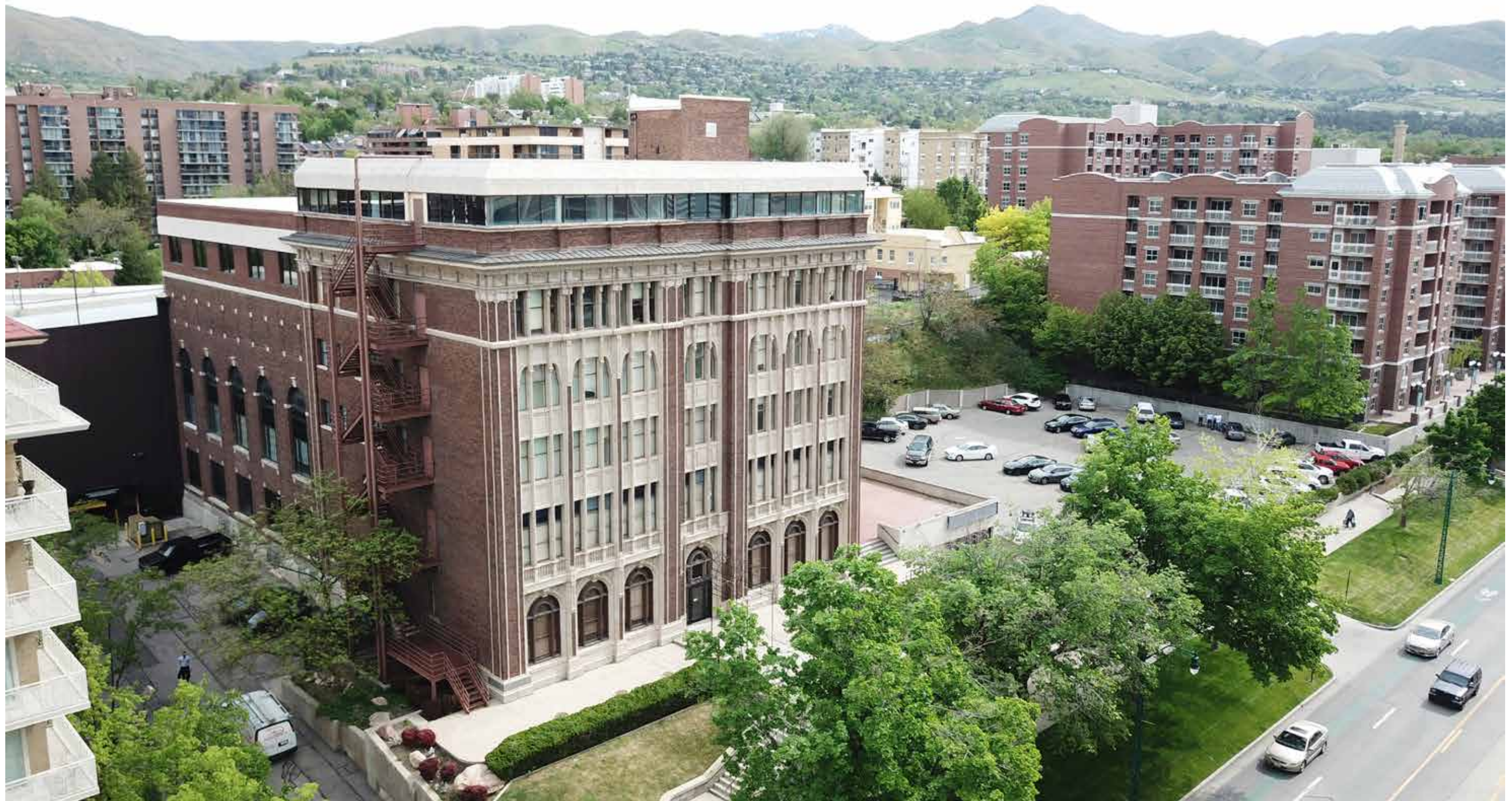
View of Existing Site
